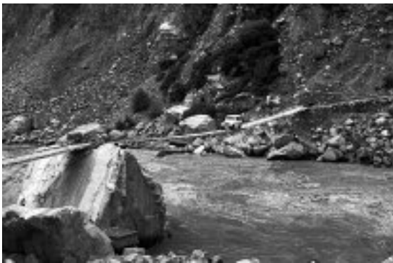
Fig. 33. Precarious suspension bridge across the Hunza river, linking a remote village with the KKH.
