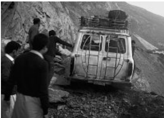
Fig. 34. Rockfalls, landslides and avalanches are a permanent danger for the KKH road track cut into the mountain slope.
