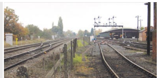
10. A view of the exchange siding taken in April 2012
