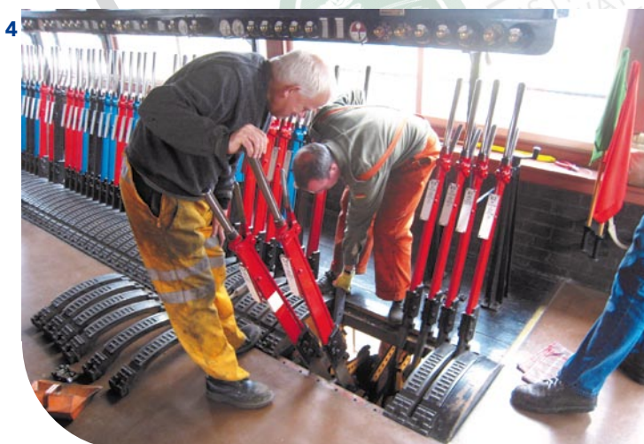
4 Levers 57 to 61 are being moved in November 2009 to become levers 56 to 60 to make space for a new (short) lever 61
