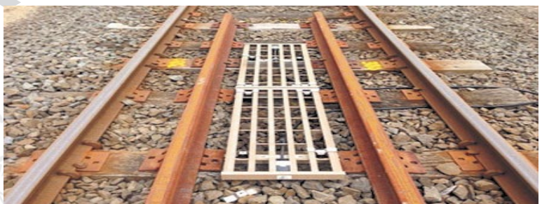
Figure 8 - #2 - Configured as Broad Gauge, Double Guard rails and TPWS Loops mounted on centre line
