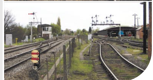
11. A view of the exchange siding taken in November 2013
