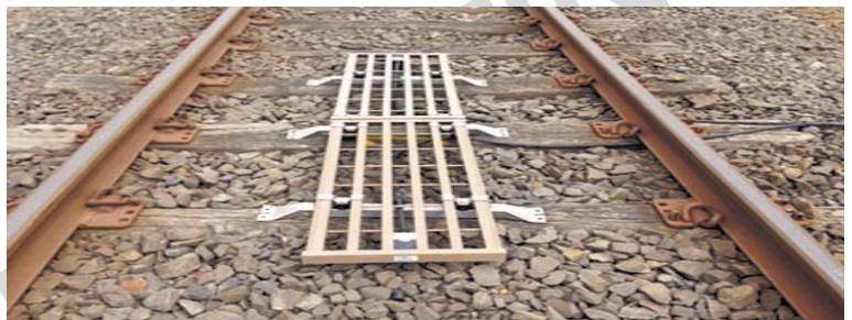
Figure 7 - #1 - Configured with no guard rail (base case and standard installation in Victoria)
