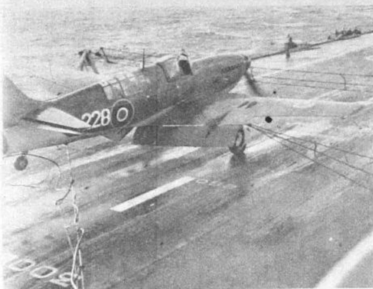
THE PILOT HAS MISSED the arrestor wire and is heading straight for the steel crash barrier . . . this is what happens, the plane is caught by the barrier but the damage is quite considerable.
