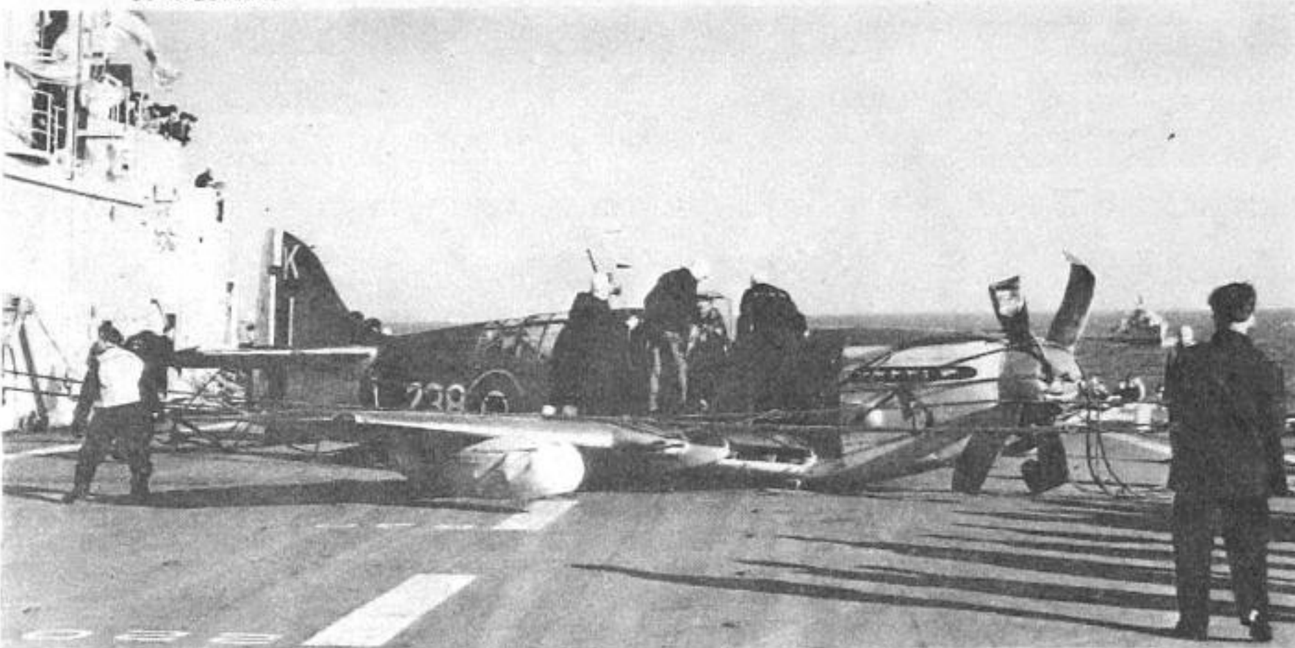
THE PILOT HAS MISSED the arrestor wire and is heading straight for the steel crash barrier . . . this is what happens, the plane is caught by the barrier but the damage is quite considerable.
