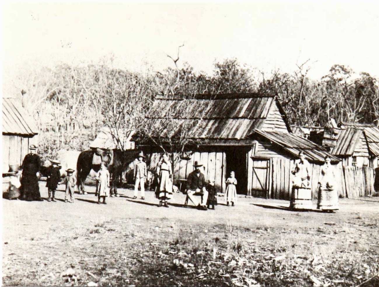
17. A settler and his family outside their bark roofed, slab walled house at Rosewood, 1880. From Trackson's Album, John Oxley Library.
