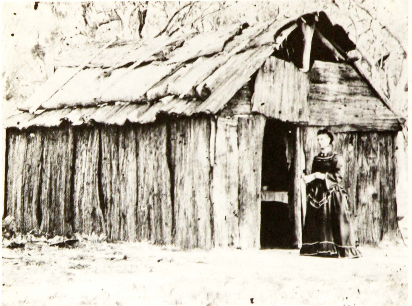
3. A hut in the pioneering days. The first house of a settler often was a simple construction with bark roof and walls. From Jack's Album, John Oxley Library.
