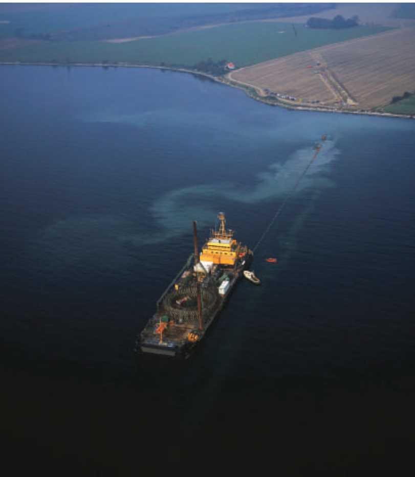
Atlantis laying the marine cable at Vantore Strand.
