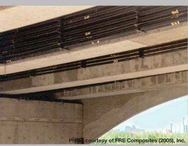
wall conduit, designated and marked as Type "XW." This conduit is suitable for use where exposed to physical damage in accordance with the NEC. It is also permitted to be used in Class I, Division 2 hazardous locations, in accordance with Section 501.10(B)(7) of the 2008 NEC.
