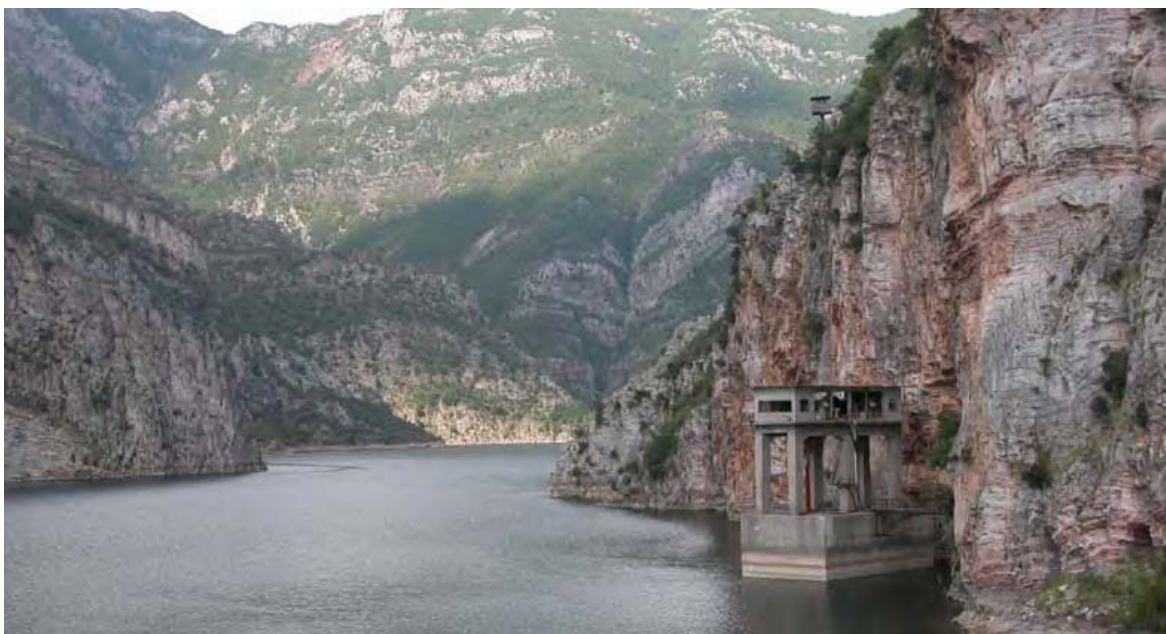
Figure 6 Intake tower of the spillway No 3
