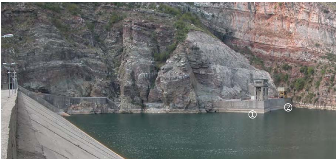
Figure 4 Gate tower of the spillway No 4 (1) and power intakes (2)
