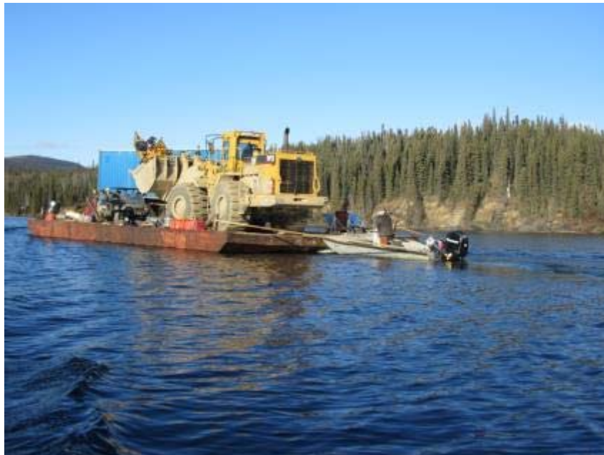
Figure 7-20: Barge Transporting Heavy Equipment on Mayo Lake
