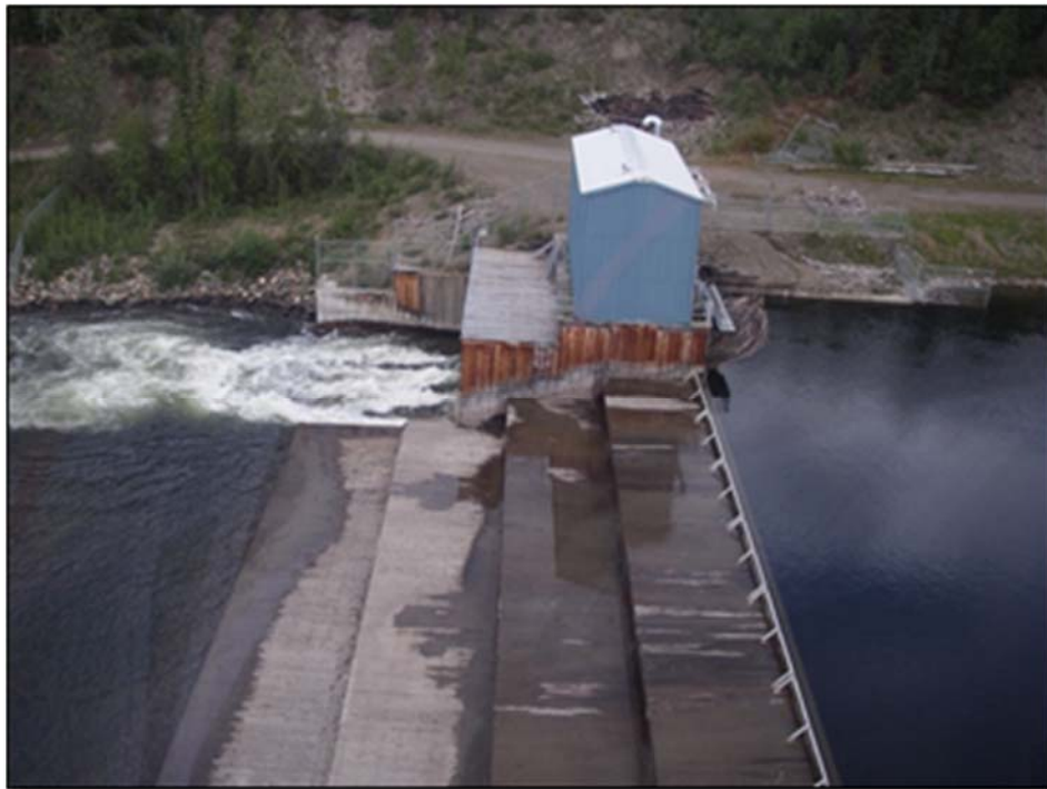
Figure 5-1: Mayo Lake Control Structure
