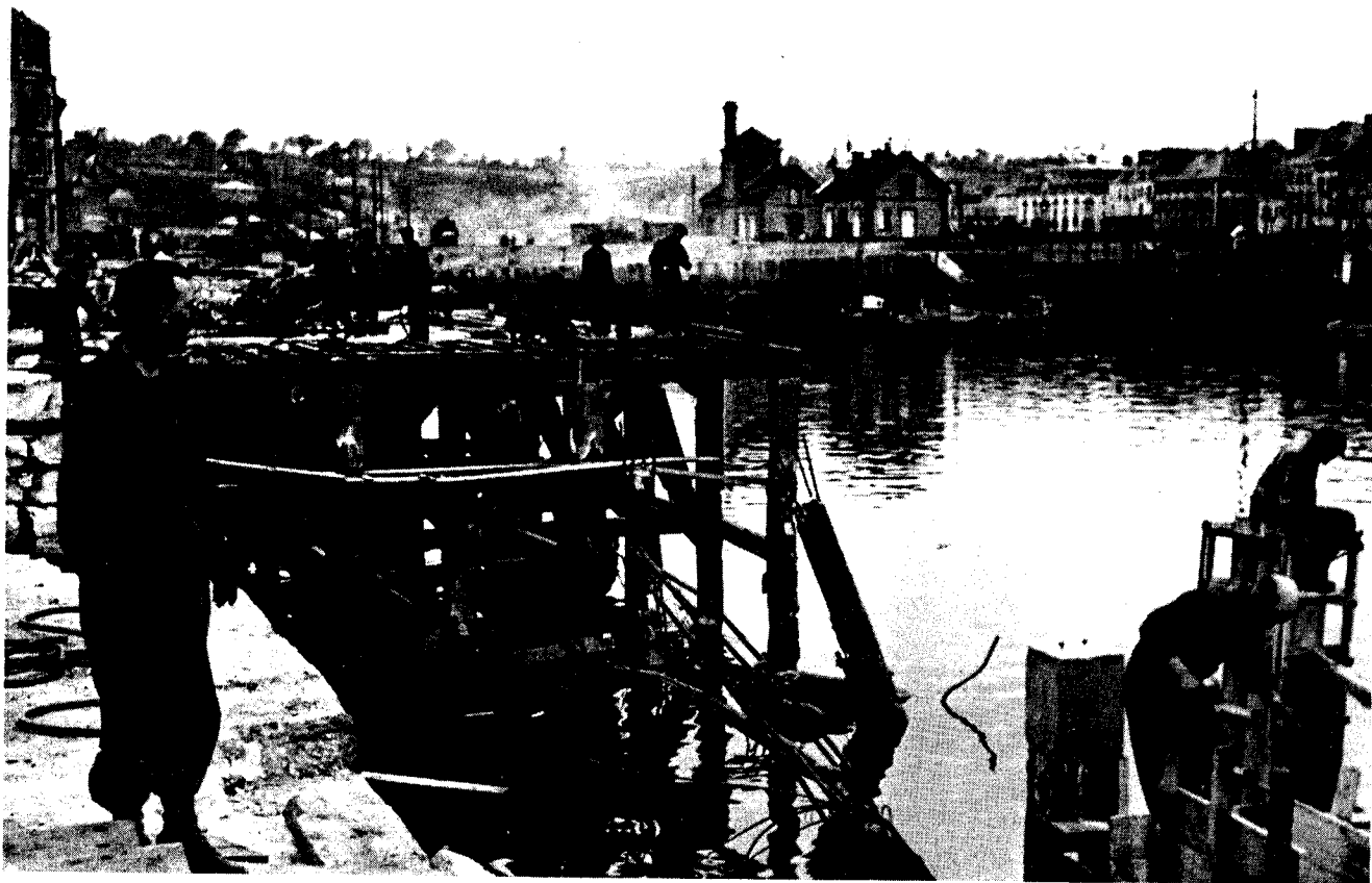
MEMBERS OF PORT CONSTRUCTION AND REPAIR GROUP building docks at Cherbourg harbor, France, July 1944.
