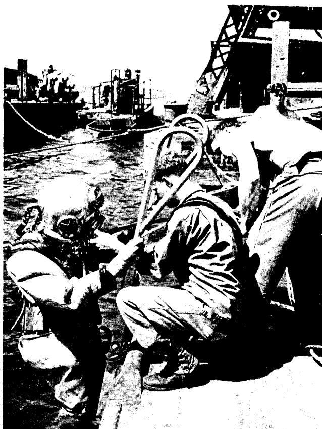
DIVER COMING OUT OF THE WATER, Camp Gordon Johnston, Fla., is engaged in underwater repair.
