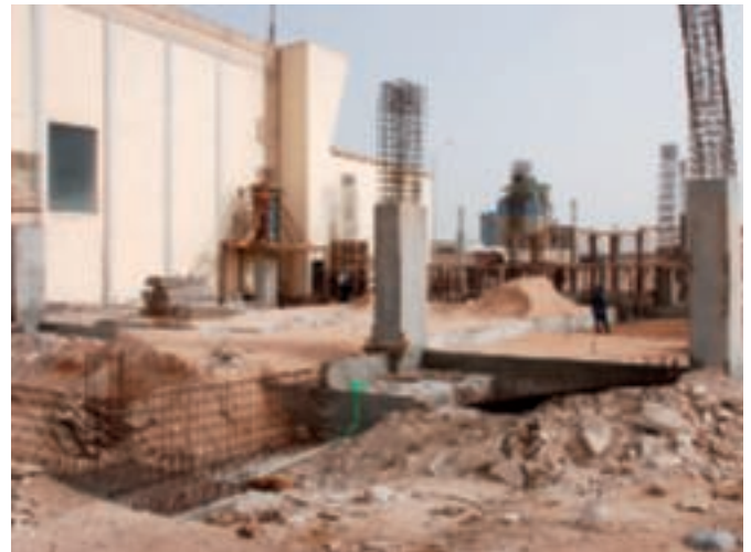
Machine hall extension.
