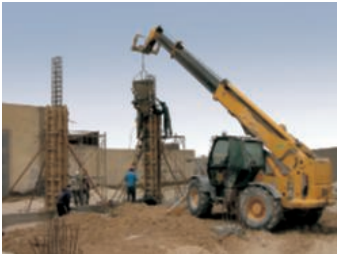
Concrete works at the fuel farm.
