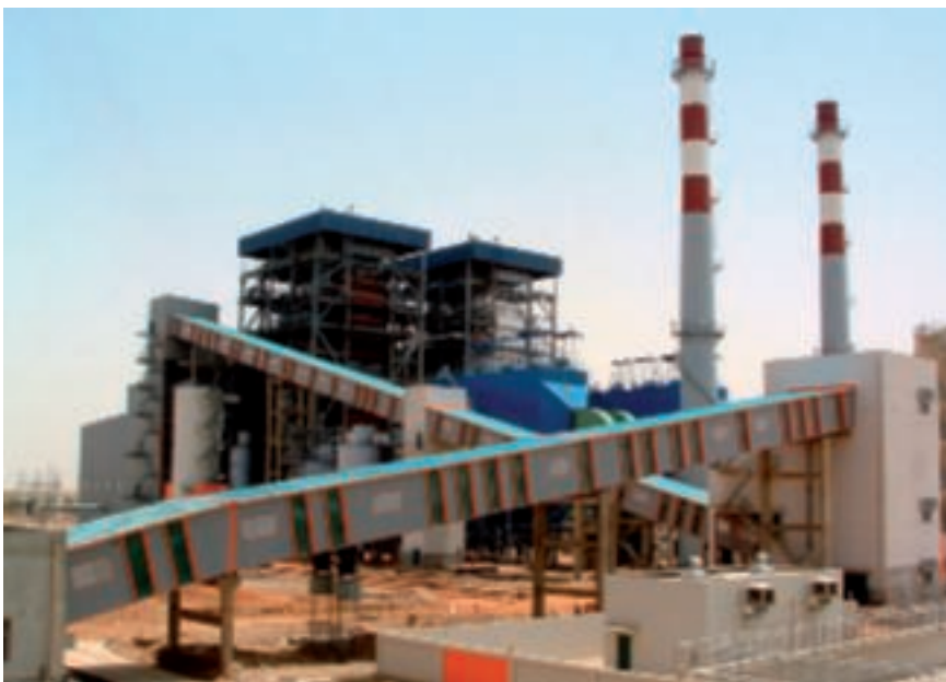
View of Garri 4 with coal transportation.
