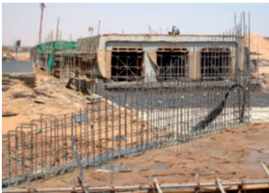
Cross-drainage culvert under construction.
