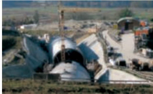
Construction pit at the west portal.
