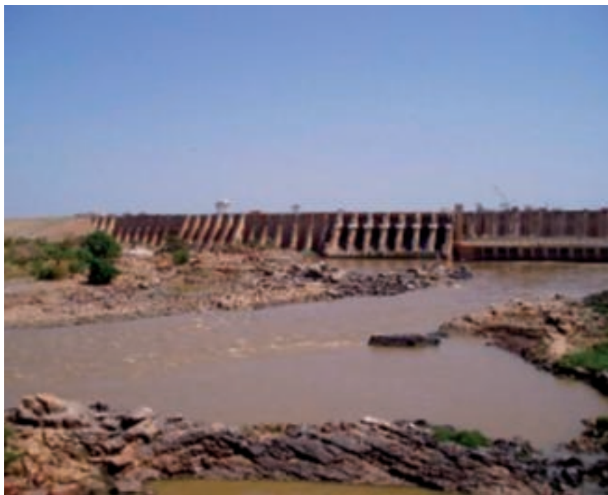
Downstream view of the Roseires Dam.
