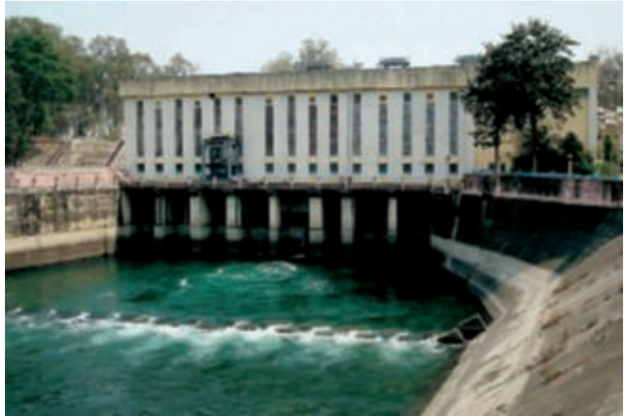
Chibro HEPP (240 MW), Ichari Dam, view from upstream.
