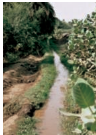
Water distribution at the lowest level.
