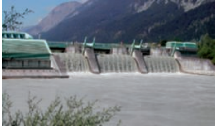
Downstream view of the barrage Langkampfen.
