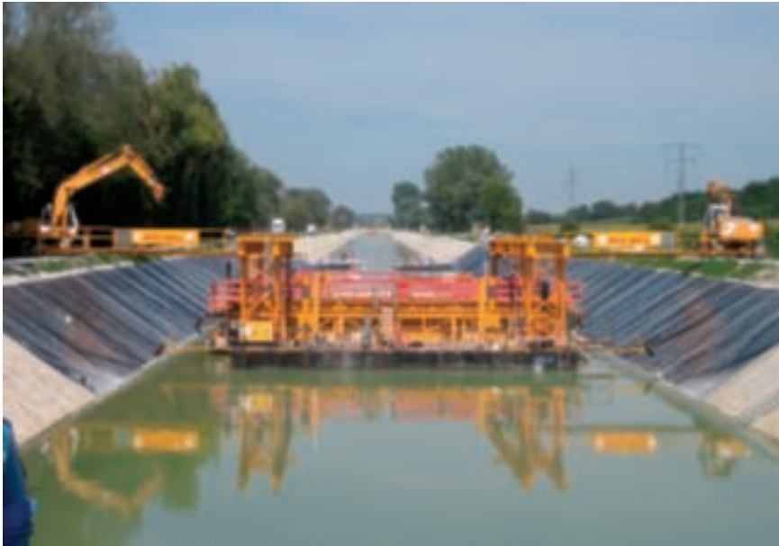
Surface sheeting and underwater concrete finisher. (Source: Hydroprojekt / Bau und Plan.)
