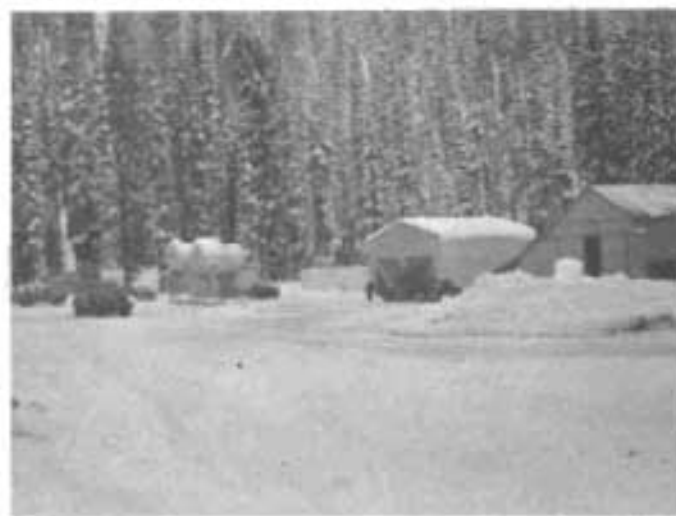
Camp, Salmo-Creston Highway—elevation 5283 ft.
