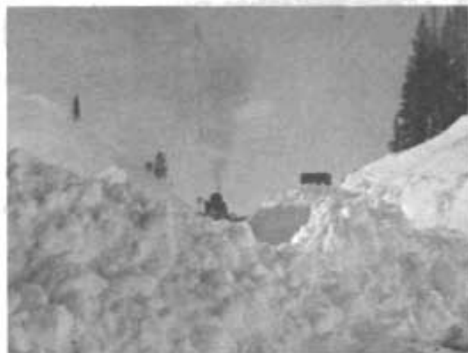
Snow slide on the Salmo-Creston Highway.
