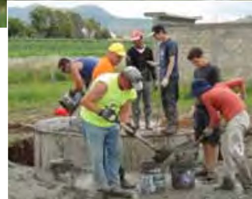
Right: Volunteers build a cistern for a rural Mazahuan village.
