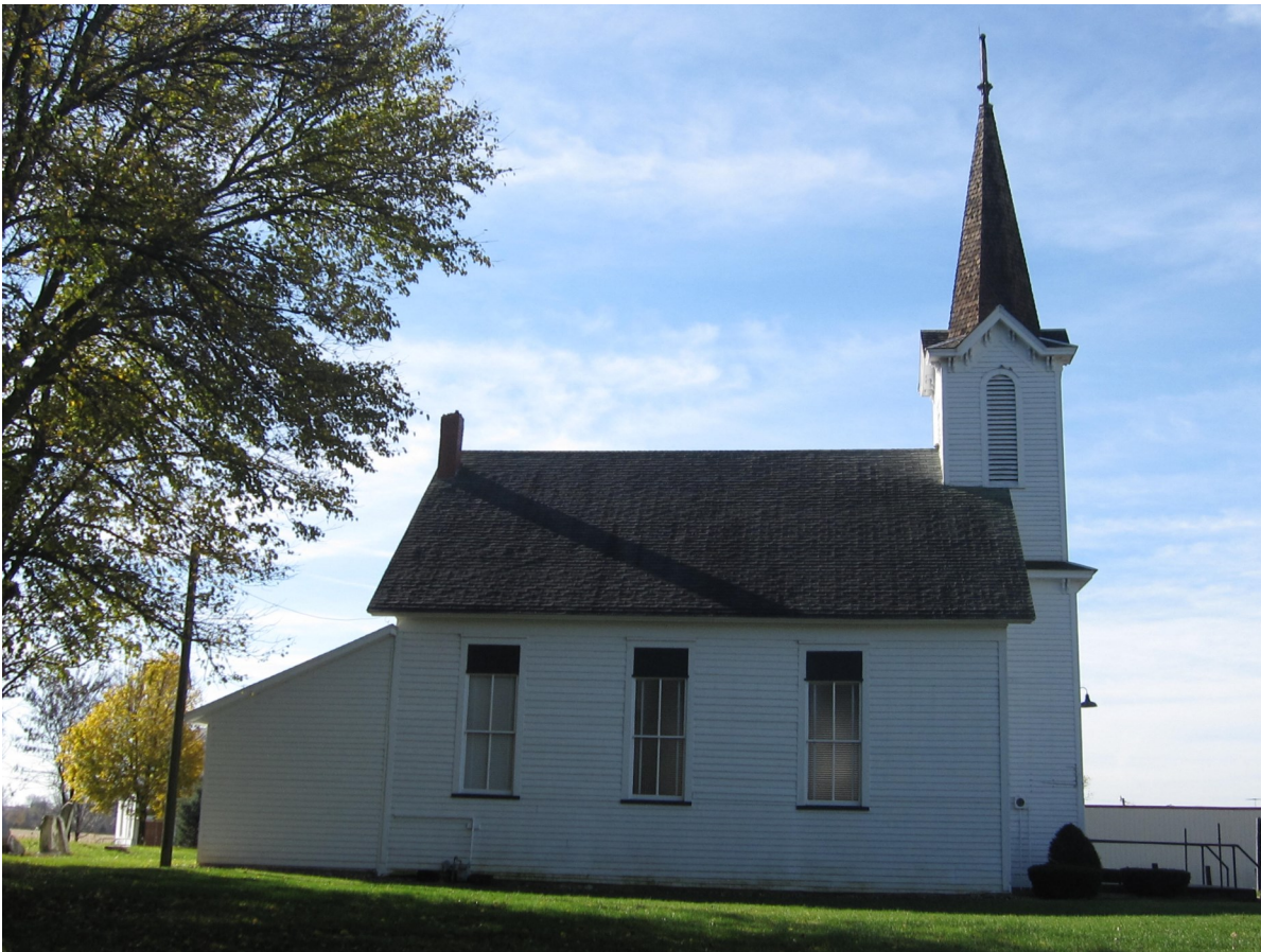
Above: Hauge Lutheran Church and the Annex read as two separate buildings.
