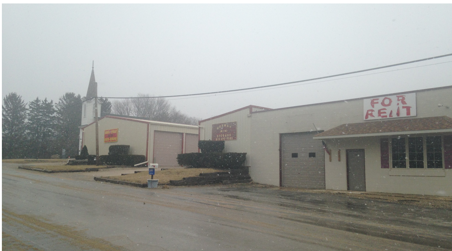
Above: Copy of 1979 Photograph showing Hauge Lutheran Church in the background. The south elevation of the church is blocked by the buildings in the foreground .
