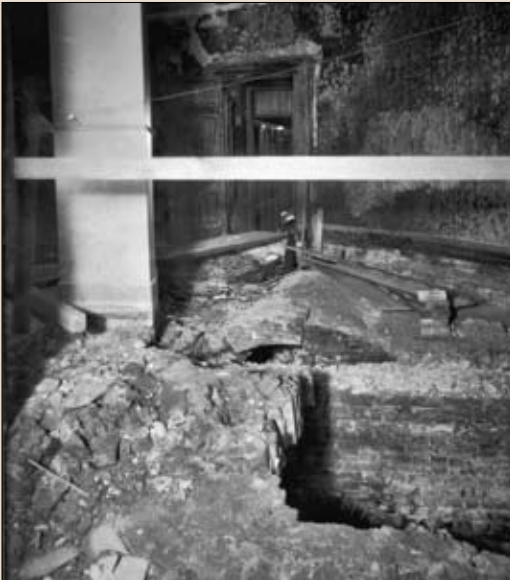
The stone floor in today's "small Senate rotunda" was blown away by the force of the gas explosion that rocked the Capitol on November 6, 1898.
