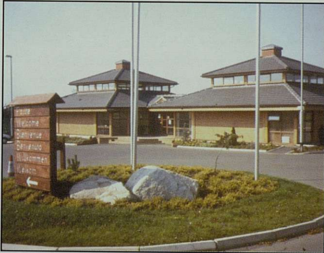
The administrative and service buildings at Camac Valley Tourist Caravan and Camping Park. (Picture by Dr. Christy Boylan)
