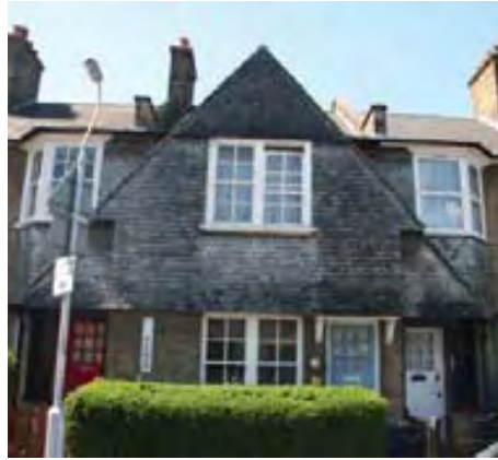
Gable containing three houses
