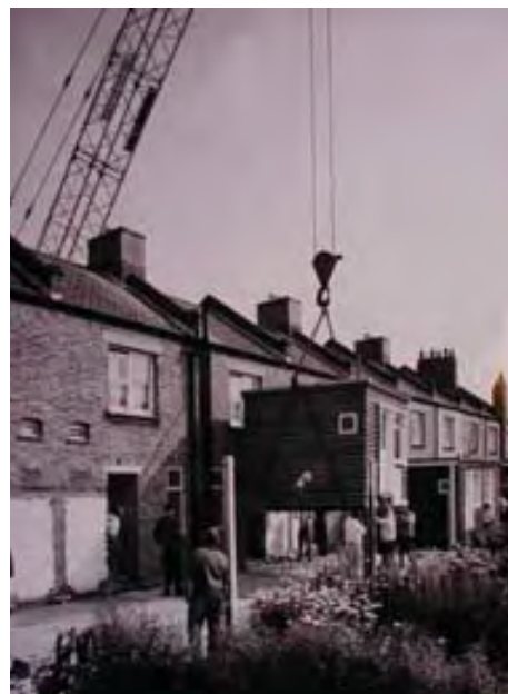
Modernisation in the 1970s: rear extensions with toilet facilities
