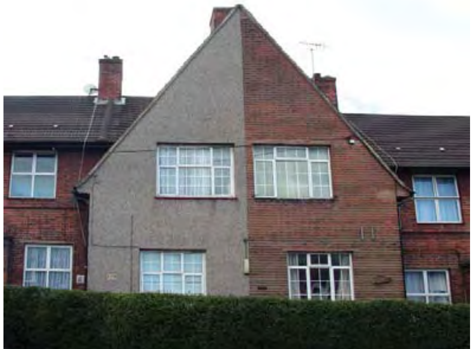
Rendering of originally exposed brick walls, disrupting the symmetry and character of the projecting gable
