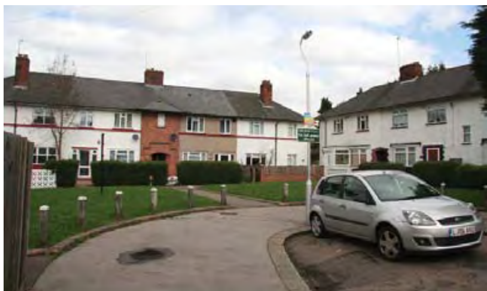
Square opening onto Northborough Road
