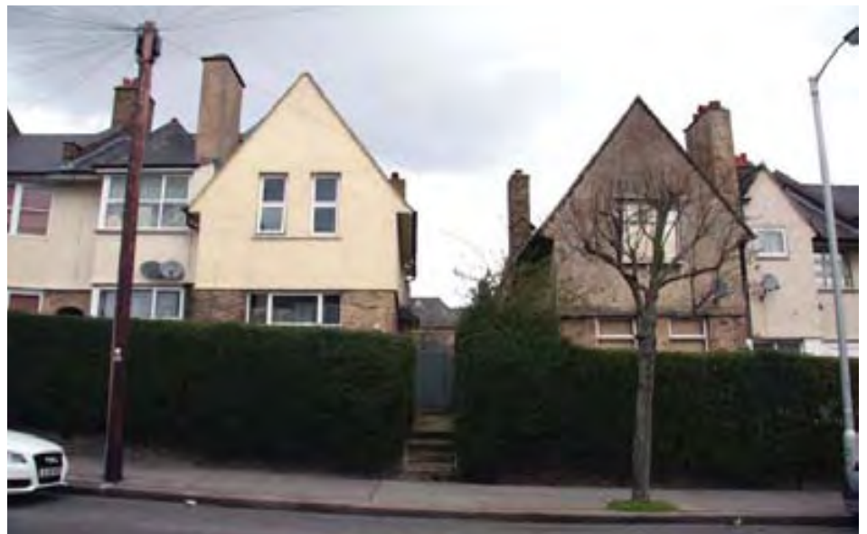
Typical spacing between the rows of terraces
