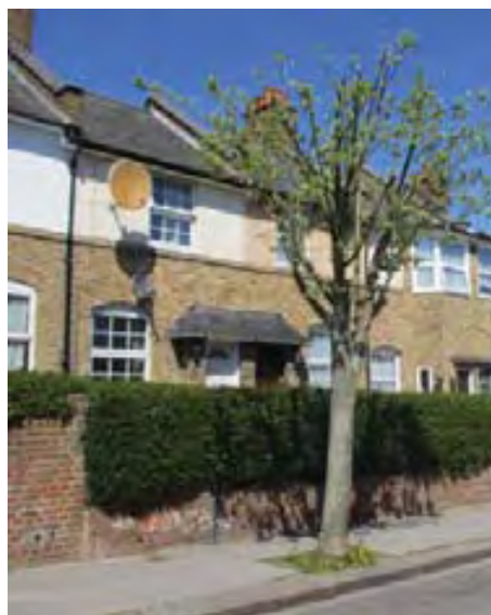
Boundaries to raised forecourts on Newlands Road
