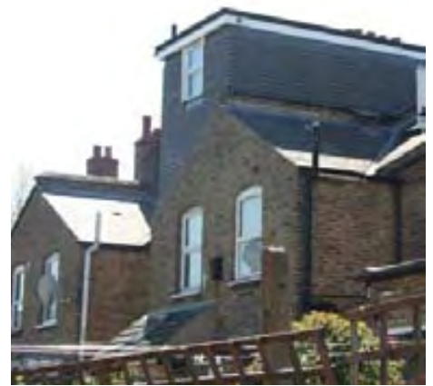
Poorly designed and dominant roof extension visible from the street
