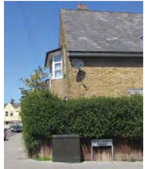
Utility cabinet and street nameplate sensitively located along the property boundary
