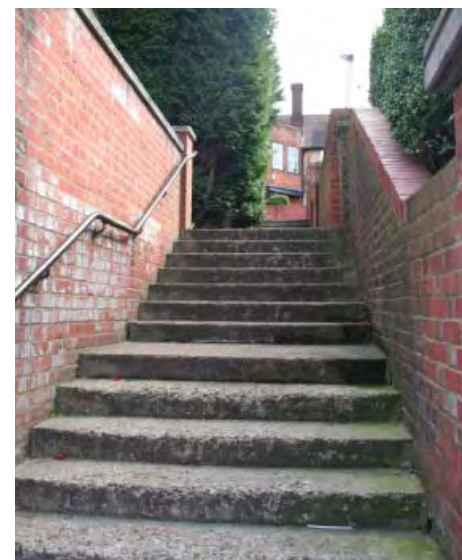
Isham Road public realm
