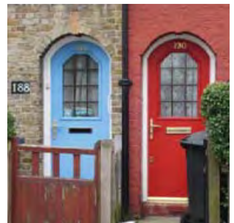
Part glazed timber doors - original design features
