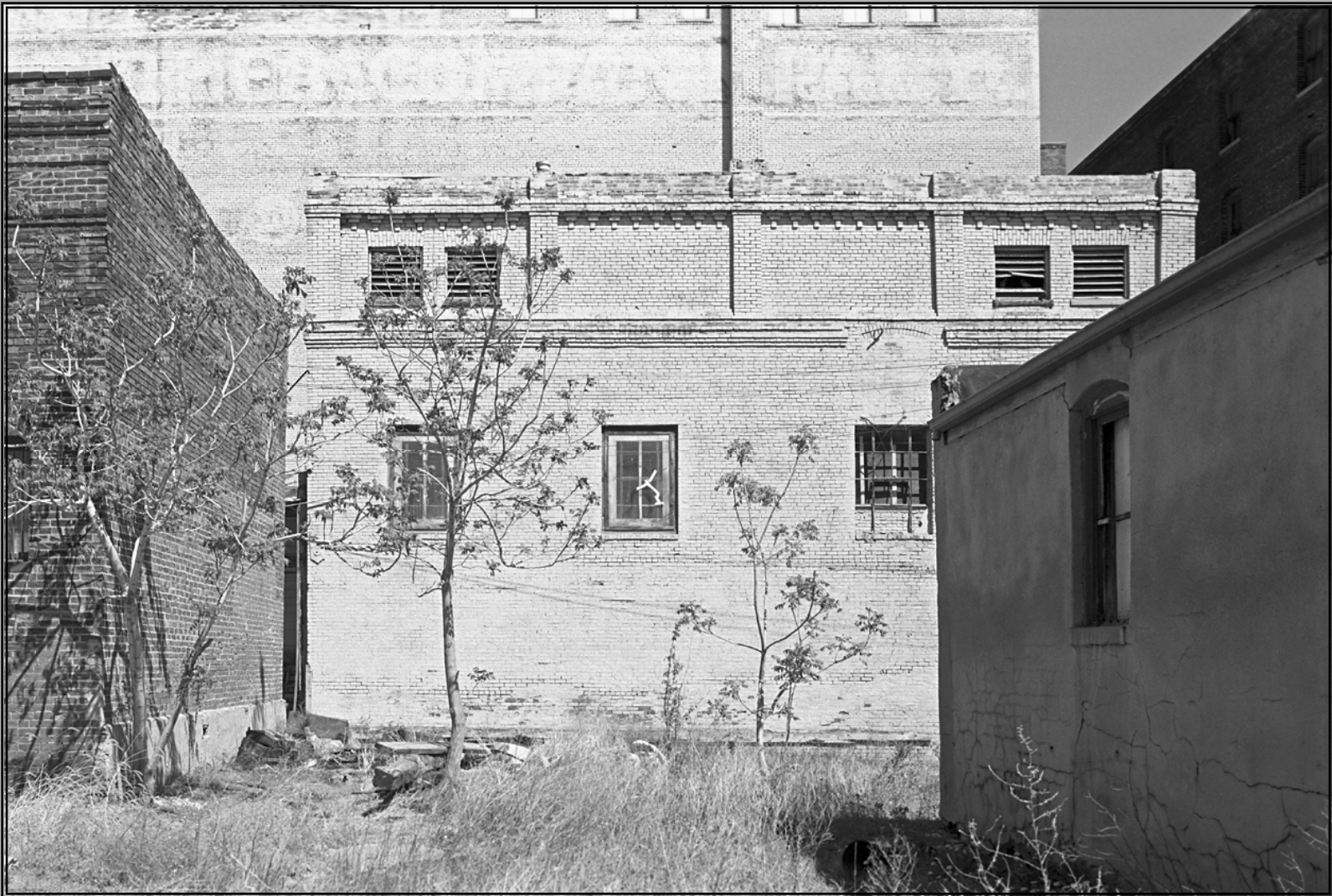
Photo 9 of 10 – ice house/beer vault, view to the east. Photo by D. Murphy, Lincoln, NE, 1978 (DM197805-D-21)
