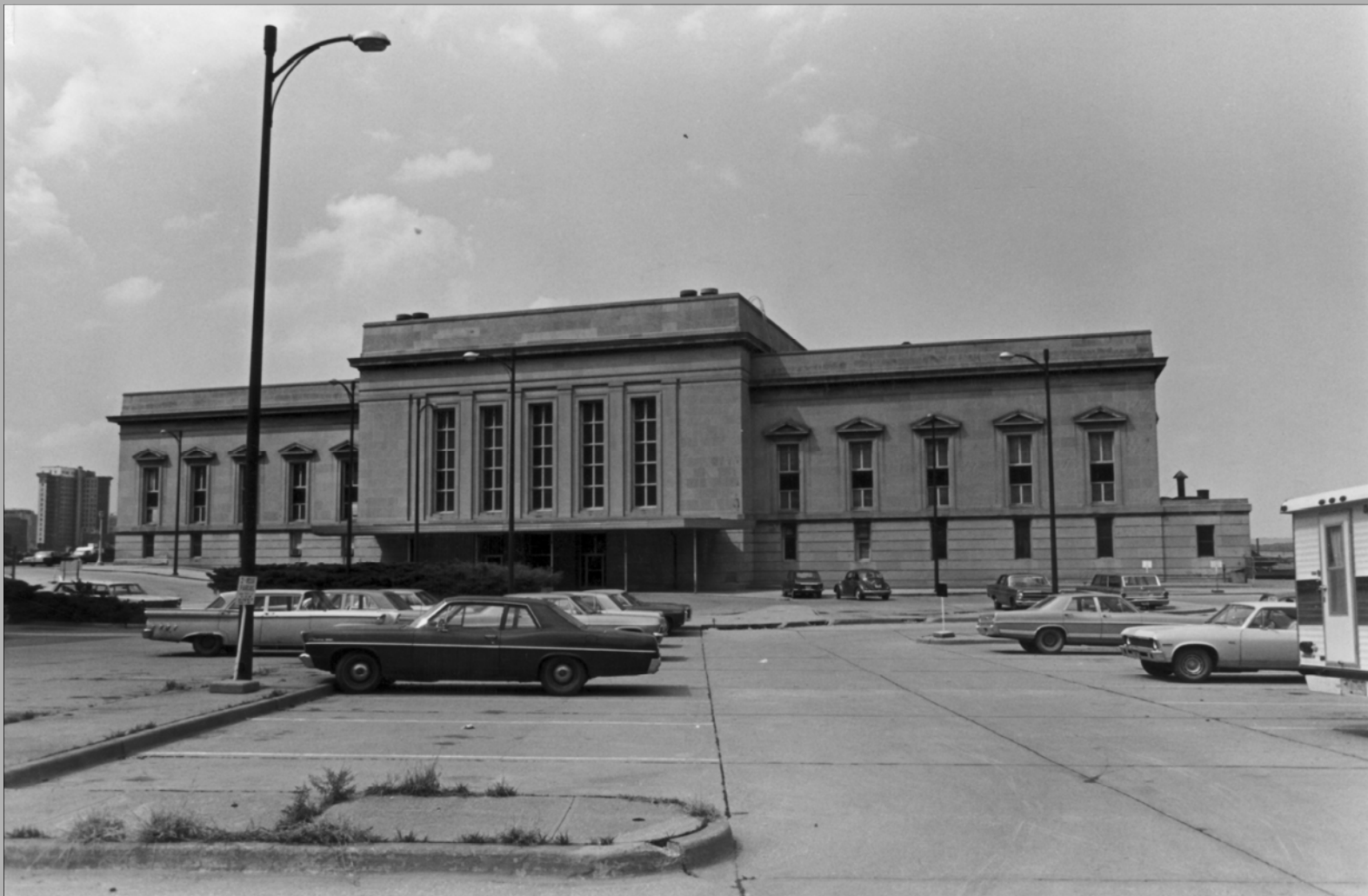
View of south elevation looking north Photo, 1971, NSHS H673.5-3081
