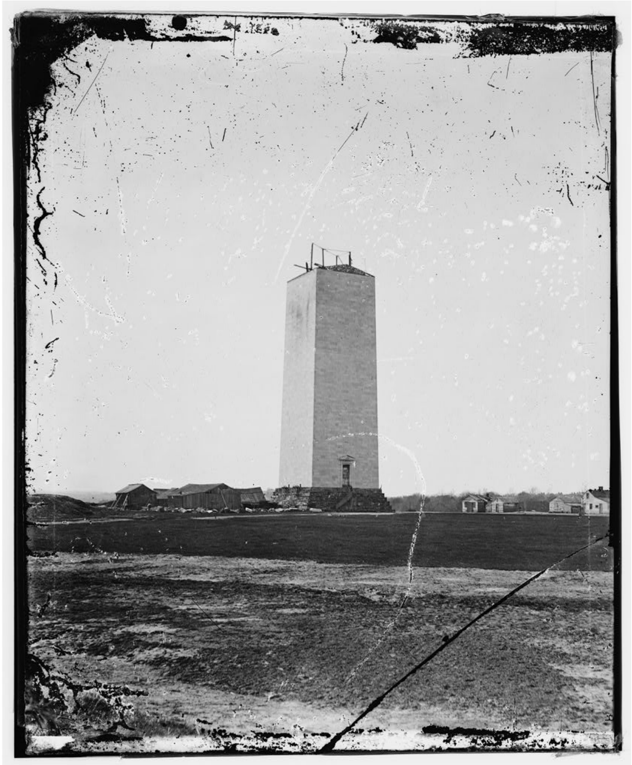
Figure 8: The Washington Monument ca. 1863 showing its unfinished state, regrading, and construction sheds (Matthew Brady, "Washington Monument as it Stood for 25 years," Library of Congress, Prints and Photographs Division. LC-BH823-2A).
