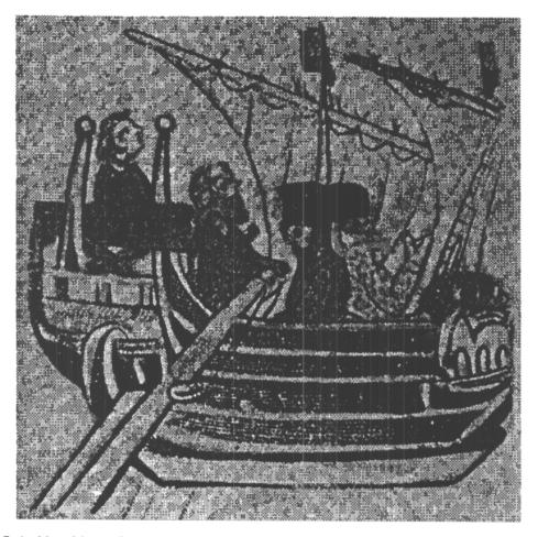
Figure 6.15 A ship with an aft-mounted quarter-rudder from the *Annales januenses*, dated 1187 (After Pryor, 1988: cover).
