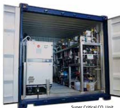
Super Critical CO 2 Unit
