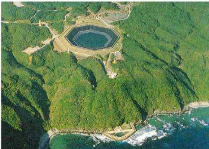
Fig. 1—Bird's-Eye View of Pilot Seawater Pumped-storage Power Plant, Okinawa Pref. in Japan. The octagonal shape shows the upper dam. The sea is the lower reservoir. The outlet of the tailrace is surrounded by tetra-pods for protection from waves.
