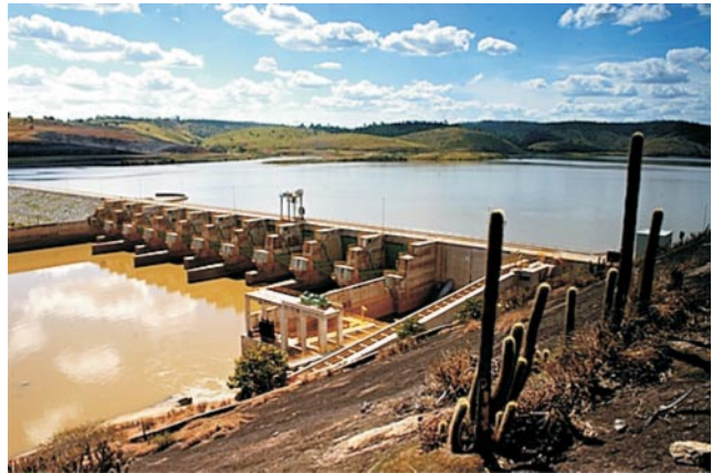
Photo 5 - Spillway Seen from the Lorena Rock on the left Bank
