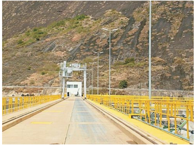
Photo 4 - The Lorena Rock along the Main Dam Axis Seen from the Spillway
