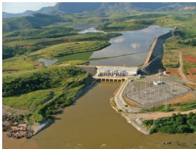
Photo 6 - The Intake/Powerhouse and Auxiliary Dam
