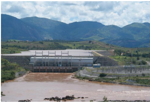
Photo 7 - Tailrace Channel with Powerhouse on the Background
