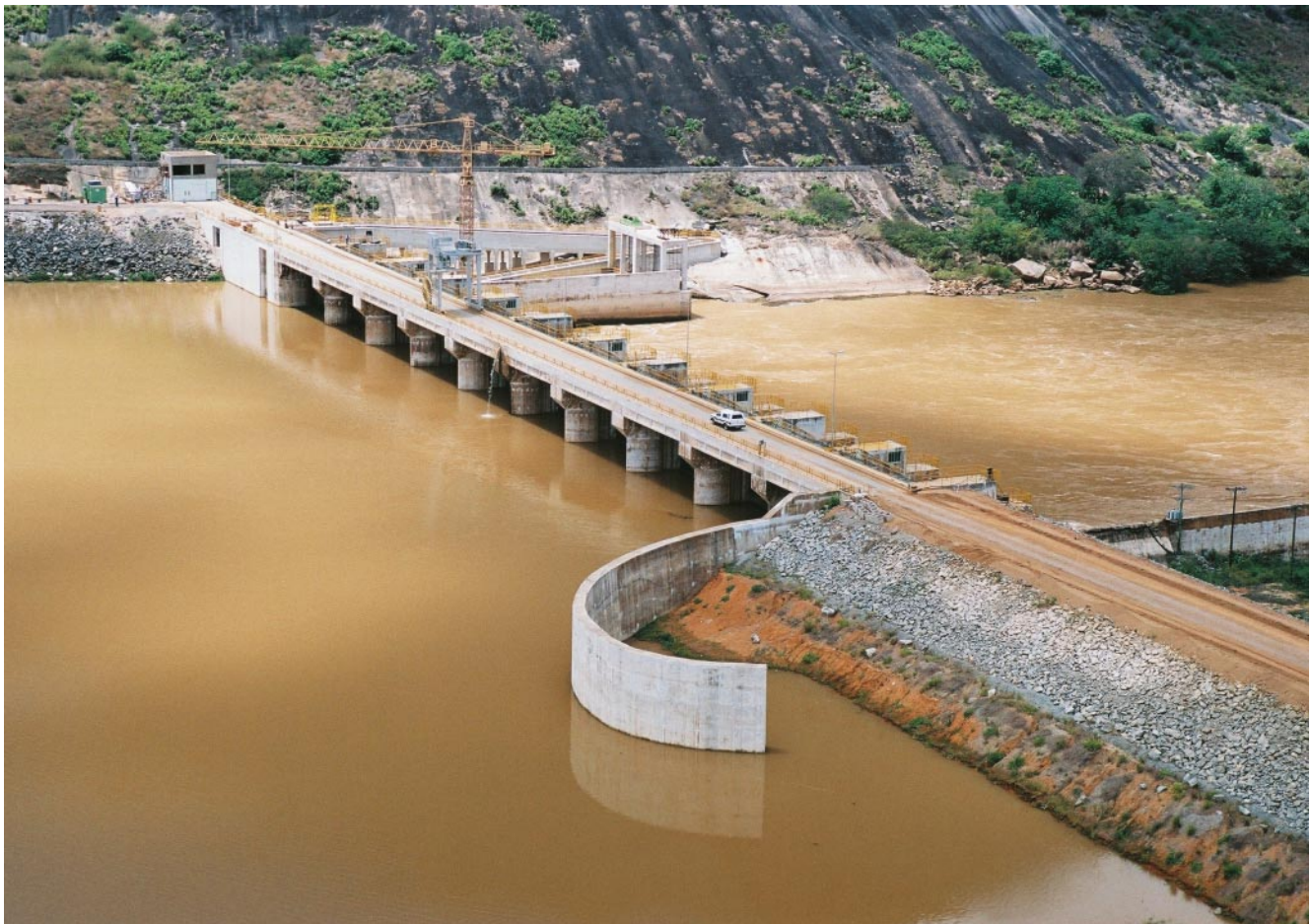
Photo 3 - Spillway and Main Dam from upstream
