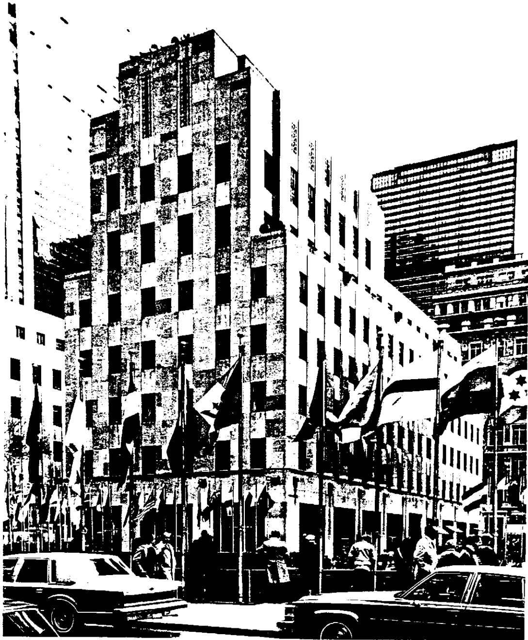
Rear Facade, View East
