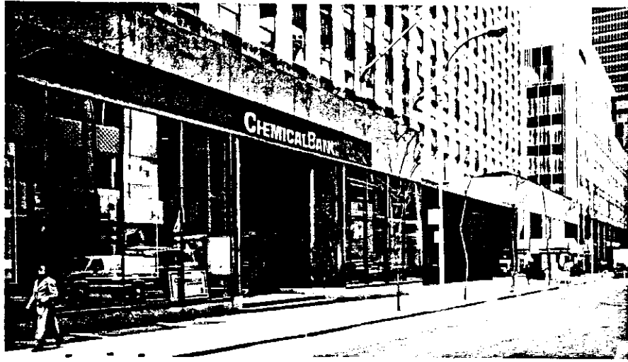
W. 52nd Street elevation, view west.
