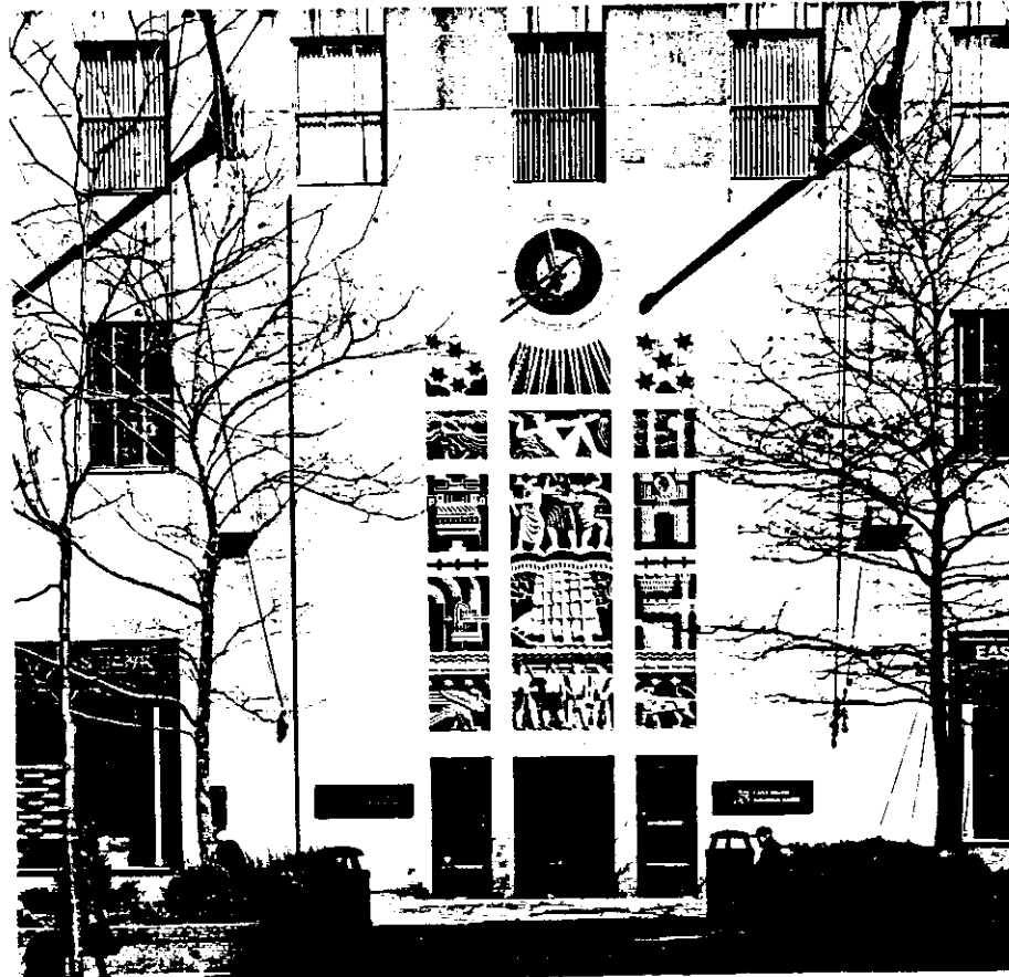
LIMESTONE SCREEN 25 W. 50th St. Entrance Lee Lawrie Installed 1935
