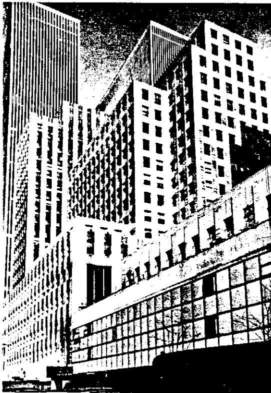
W. 48th Street, view west. Original building and perpendicular extension. Former Eastern Airlines Building at right.
