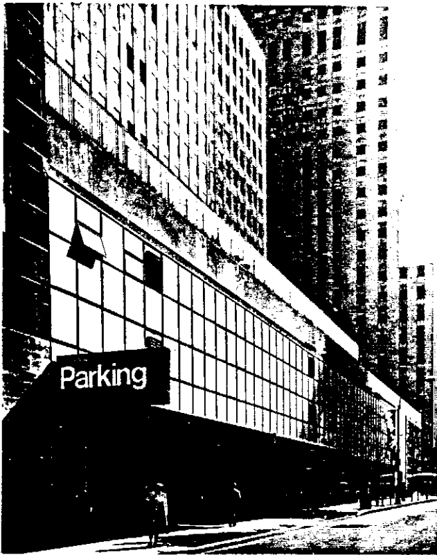
West 48th Street elevation, view east.
