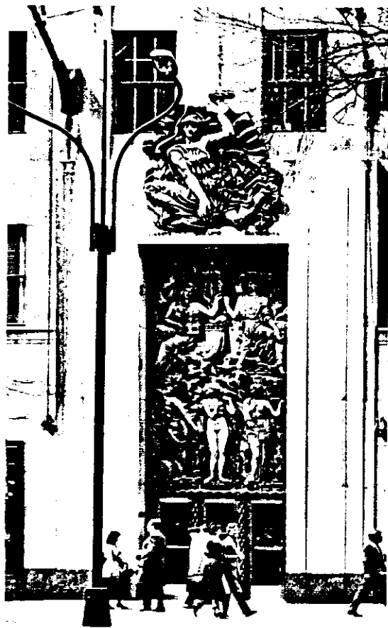
BRONZE PANEL & LIMESTONE CARTOUCHE Main Entrance Alfred Janniot Installed 1934
