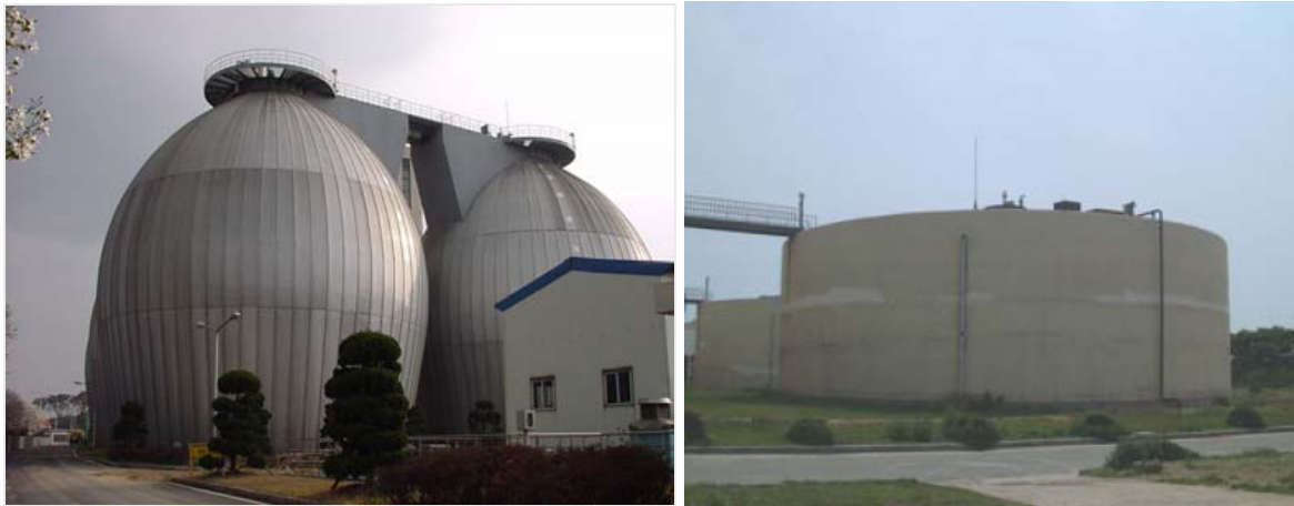
FIG. 101. View of typical oval(left) and cylindrical (right) sludge digesters
