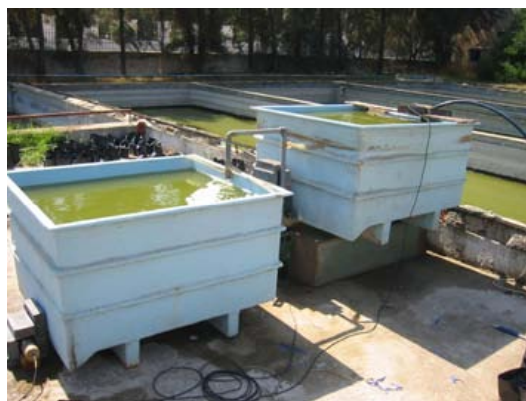
FIG. 135. Pilot scale system of two tanks in series where water moves by gravity
