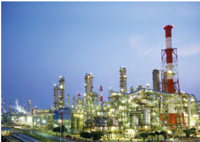
The Greenhouse Gas Reduction and Management Act has ushered Taiwan into the era of low-carbon emissions. Photo shows night view of the Linyuan Petrochemical Plant in Kaohsiung (Courtesy of CPC Corp., Taiwan)
