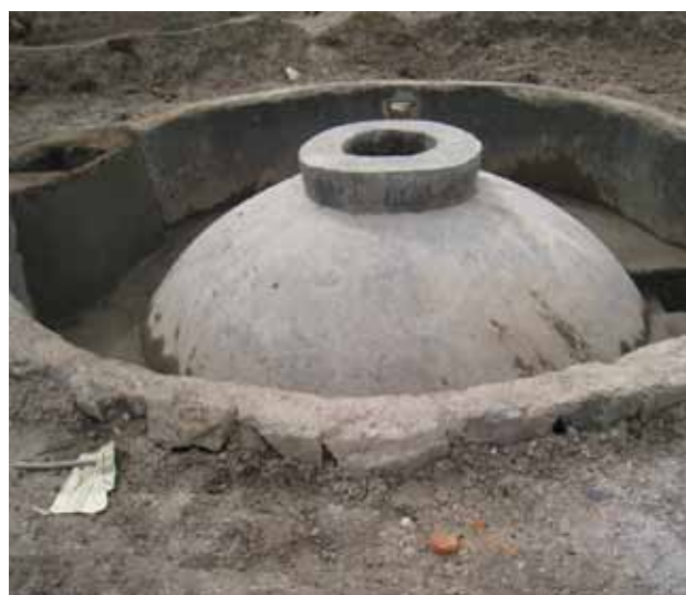
Figure 4. Biogas latrine facility in Kibera, Nairobi, Kenya, exploited by, for example, Umande Trust ( www.umande.org ). Left: multifunctional building with ground floor: latrines and showers; first floor: meeting rooms, offices, kitchen; top floor: open side for community gatherings, for example. Right: subterranean biogas digester underneath the multifunctional building.
