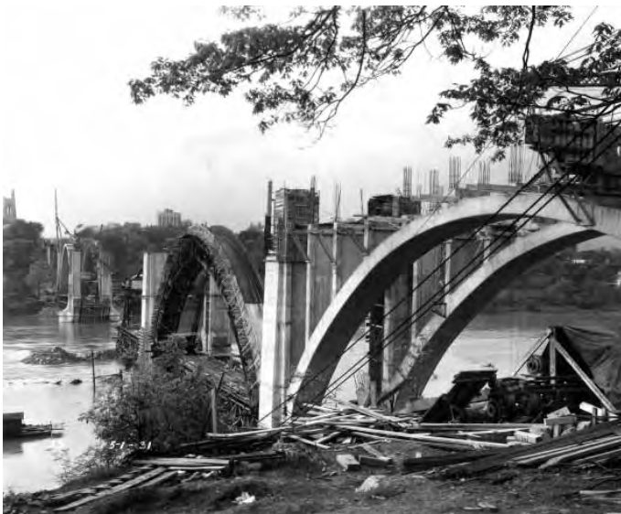
Henley Street Bridge, under construction
