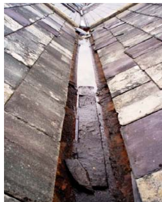
Crate of new Welsh slates ready for use. Detail of cast-iron gutter and roof valley before & after repair.
