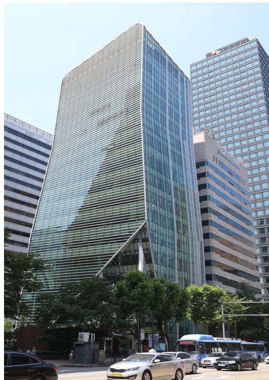
The Seoul Global Center, South Korea's largest one-stop support service center for foreigners, opened on June 21, 2013, in downtown Seoul. The U.N. Human Rights Office is located in the 19-story building, with four floors underground, which houses an immigration office, international conference facilities, the Seoul International Resolution Center and banking services. (Yonhap)
