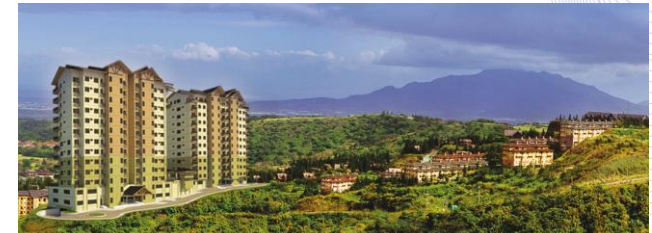
Construction of Woodridge Place's Mahogany and Linden buildings
