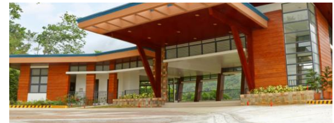
The Aspenhills Village Hall
