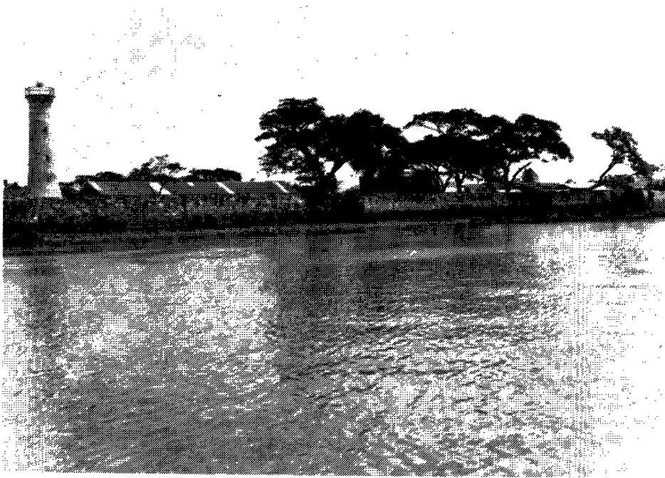
SOUTH WALL - SEAWARDS - KUALA KEDAH FORT
