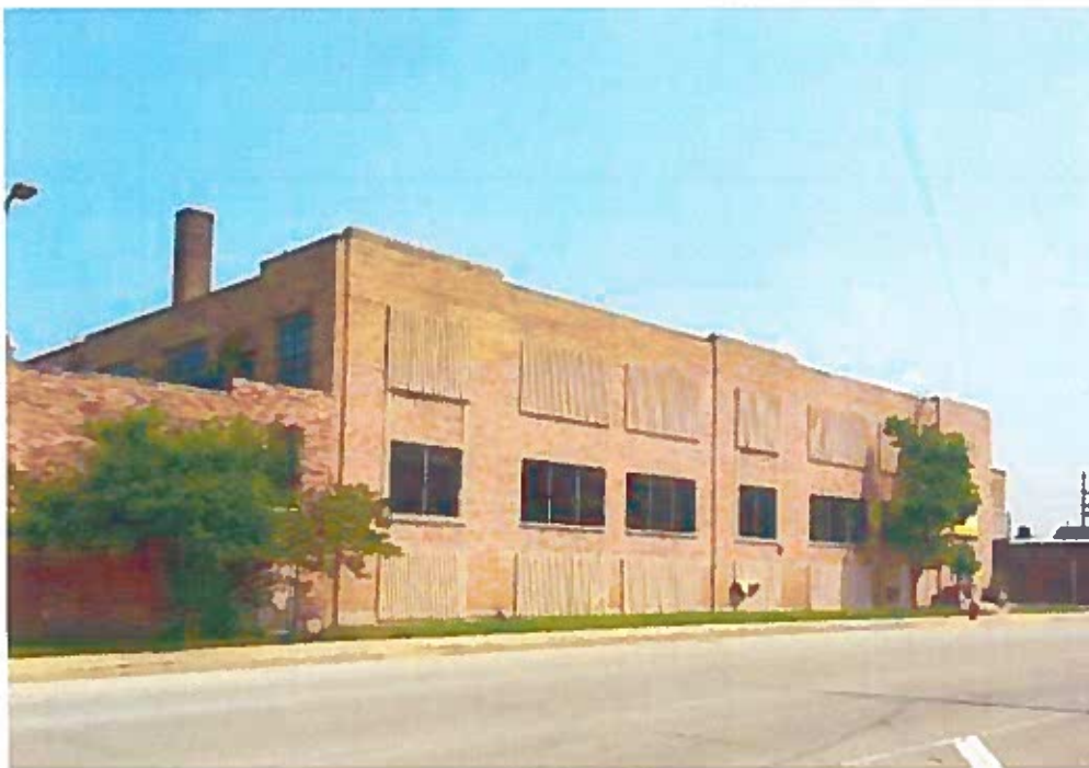
Fig. 12 – Current view of 227 S. River St. – East elevation
