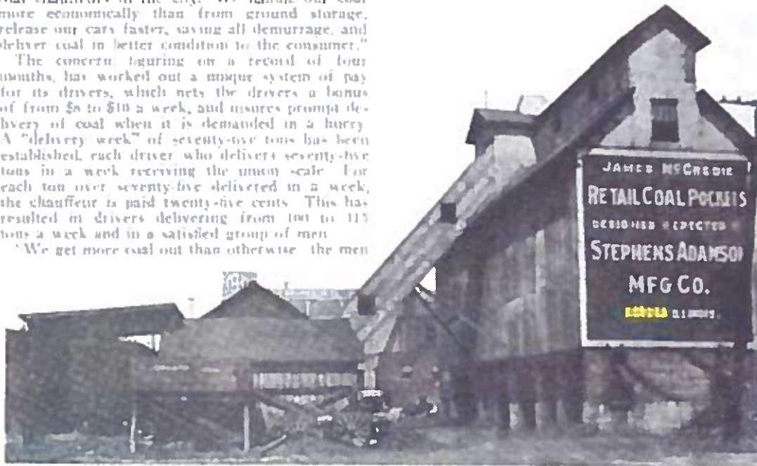
Fig. 5 – McCredie Coal Pocket (erected 1916, not extant) with the International Harvester building at 251 S. River St. visible in the background.
