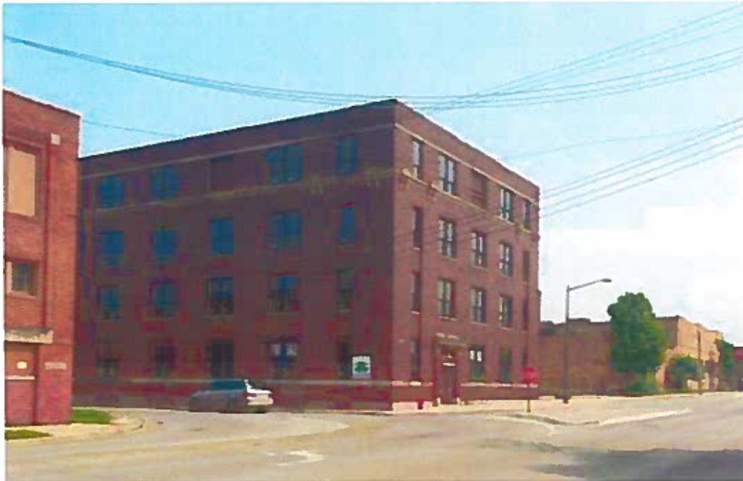
Fig. 9 – Current view of 251 S. River St. – South and East elevations
