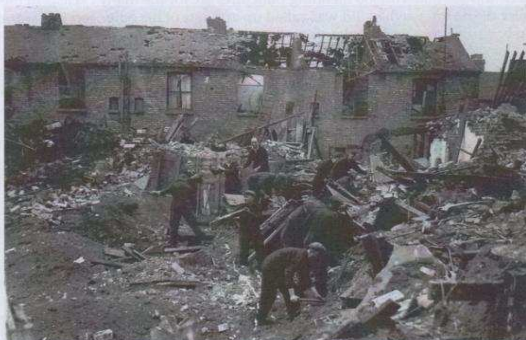
Bomb damage in Sculcoates Lane, May 1941. Hull Daily Mail.
