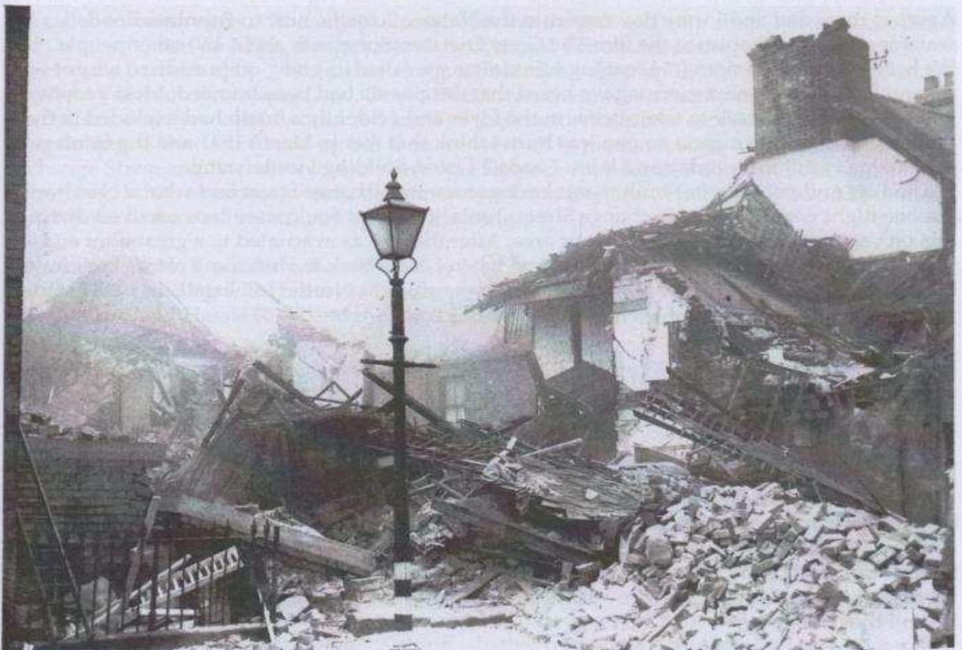
Houses in Cave Street off Beverley Road, completely destroyed. Hull Daily Mail.
