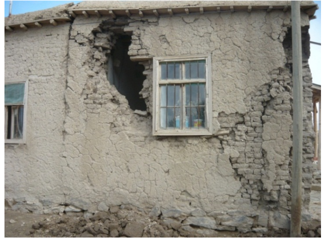
Fig. 11. Wall opening close to the building corner (Güveçli village, Van).
