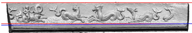
Figure 8. The main front of the frieze with the misalignment between the upper plane (red) and the cornice (blue)
