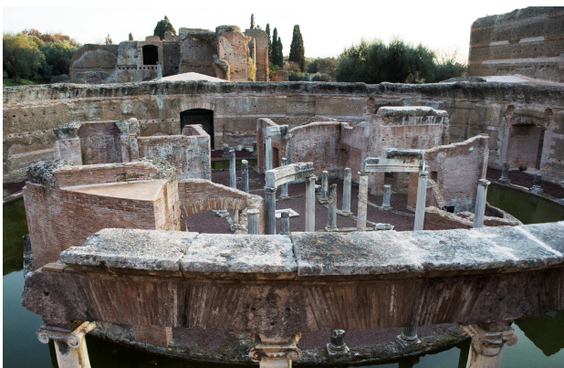
Figure 1. Overall view of the Maritime Theatre
