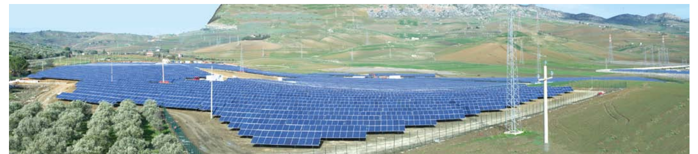
Photovoltaic power generation plant in a suburb of Ciminna, Sicily, Italy
