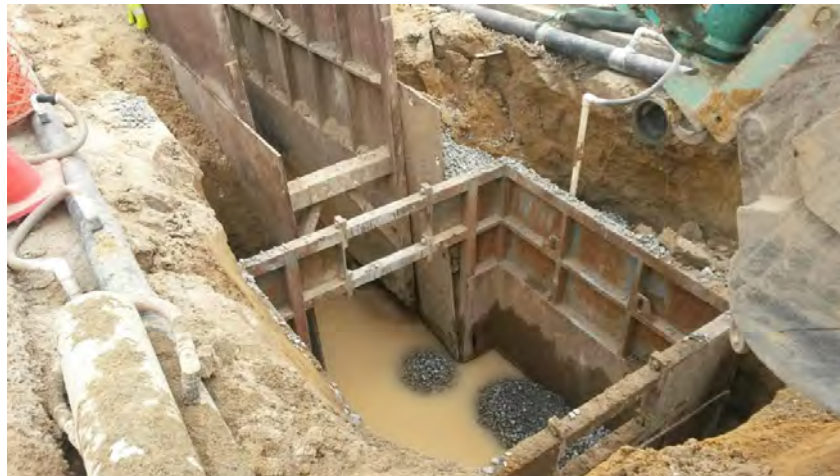
George Street Groundwater Dewatering
