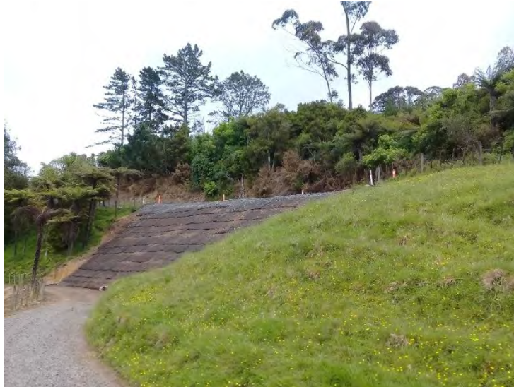
Bluff Road underslip repair
