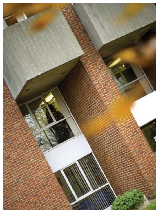
The Mantell Building, home to the International Study Centre
