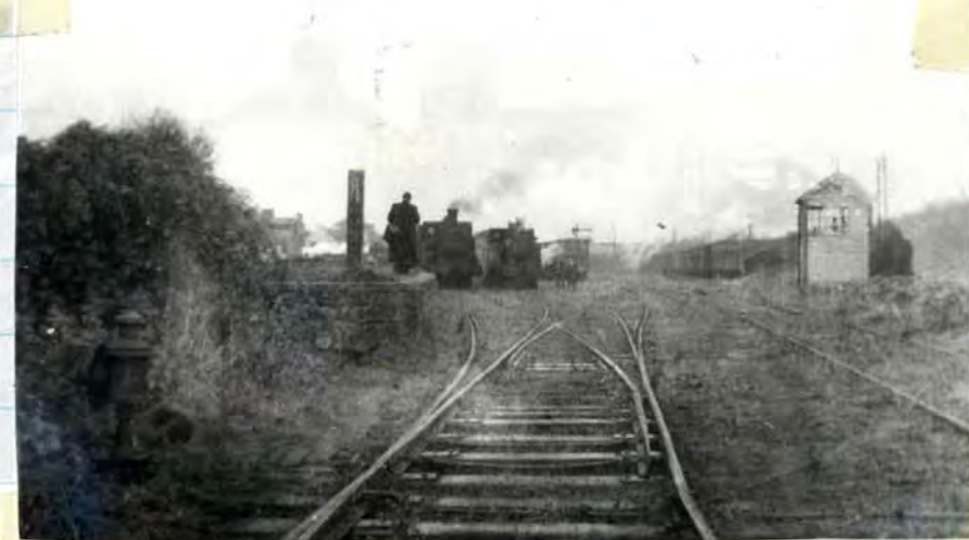
GENERAL VIEW OF MACROOM STATION ON CLOSURE DAY.
