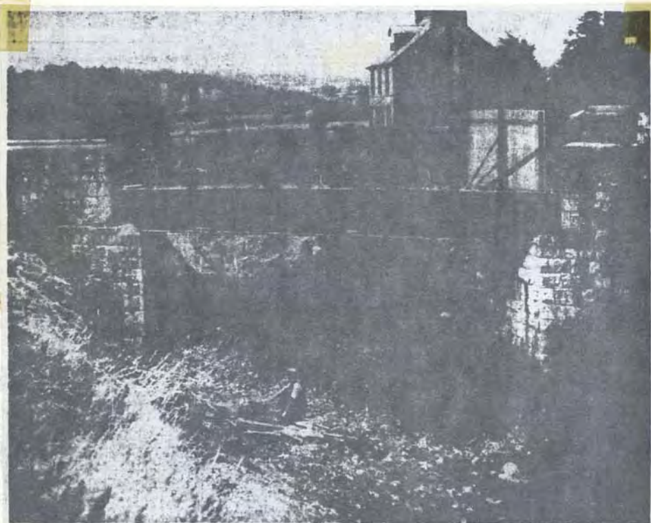
The railway bridge at the junction of Capwell Road and South Douglas Road, Cork, which is being dismantled by C.I.E. The railway outting is being filled in to carry the roadway. - ("Examiner" photo).
