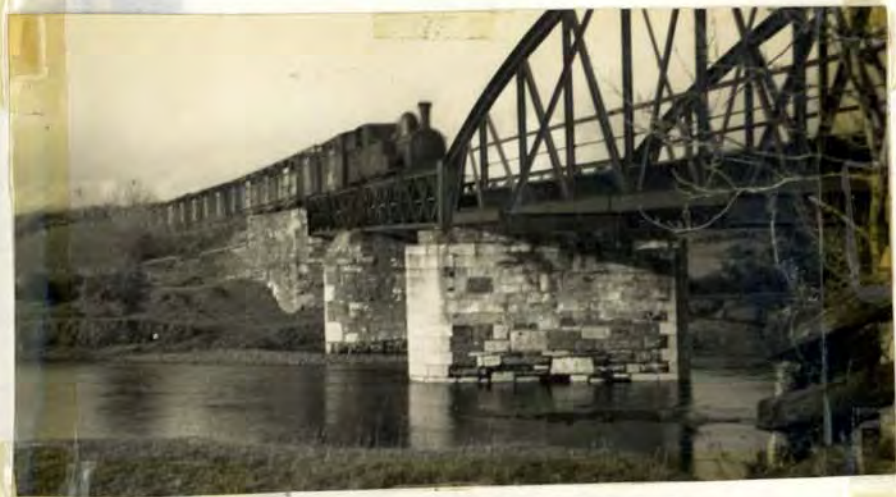
SECOND SPECIAL APPROACHING LEE VIADUCT. (WALTER MR. GRATH)
