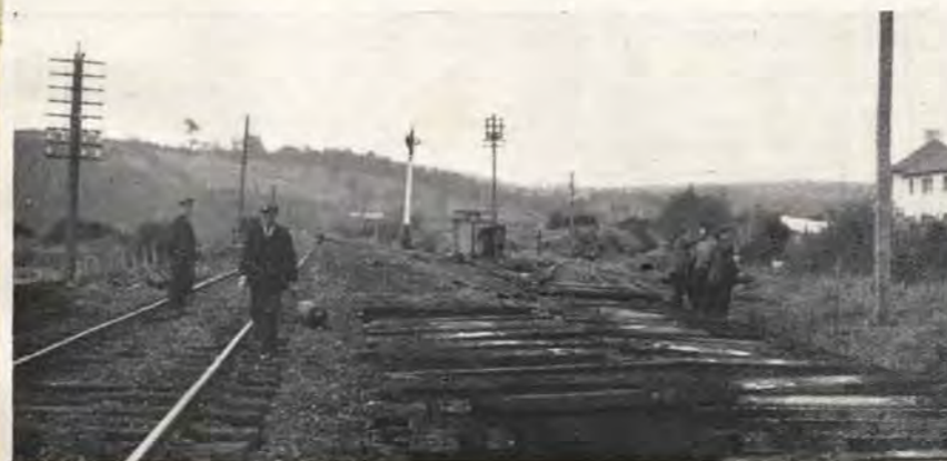
Demolition gang removing the junction between the Macroom and Bandon lines, near Cork, on November 27, 1955
