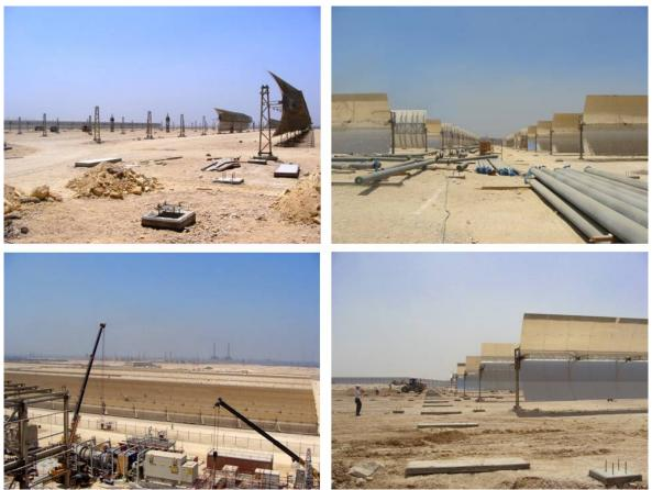
**Figure 6-2 Collector Installation Progress**
