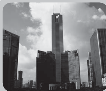
Guangzhou-Zhongtian Square Guangzhou Branch
