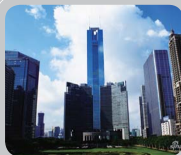
Guangzhou-Zhongtian Square Guangzhou Branch
