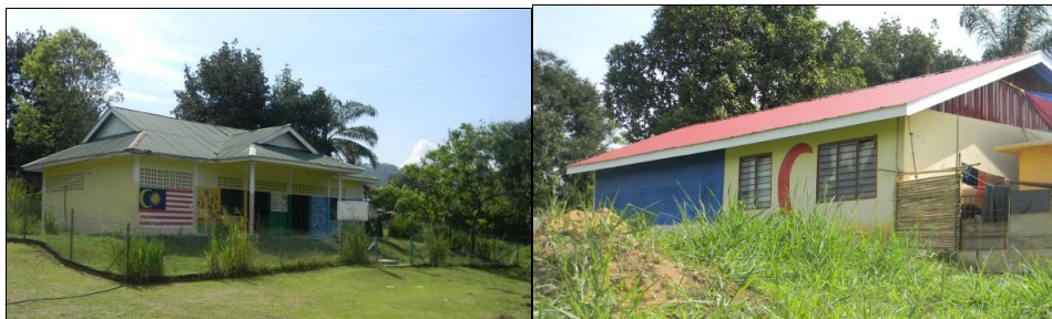
Fig.3. Infrastructure at Kampung Sungai Tiang
