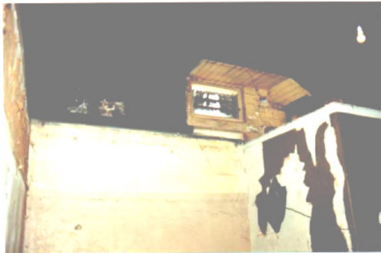
Ceiling in Room 0.6
