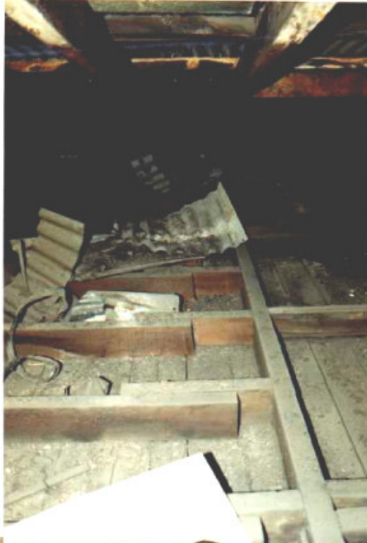
103.5 Extended ceiling joists over Room 1.4a
