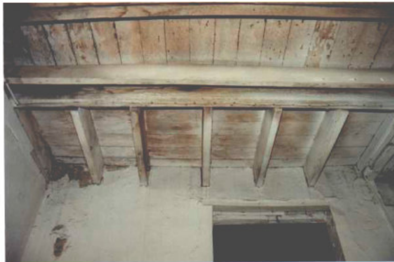
Closed over opening of the original stairs Room 1.6
