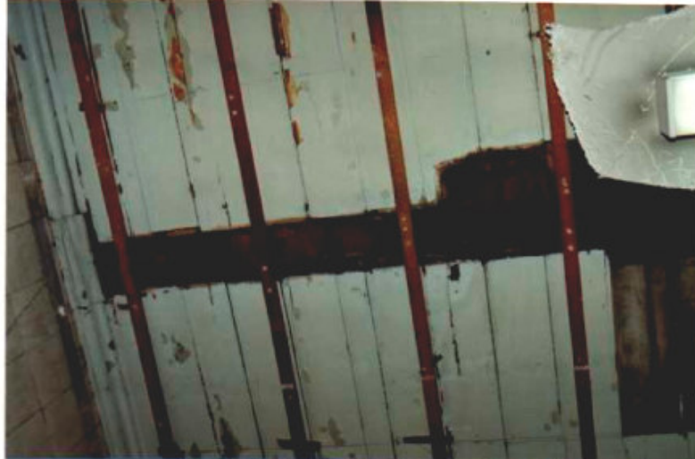
103.1 Removed partition wall showing original paneled ceiling Room 0.3
