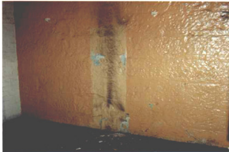
Impression of the roof line of rear room in the stone wall Room 1.4
