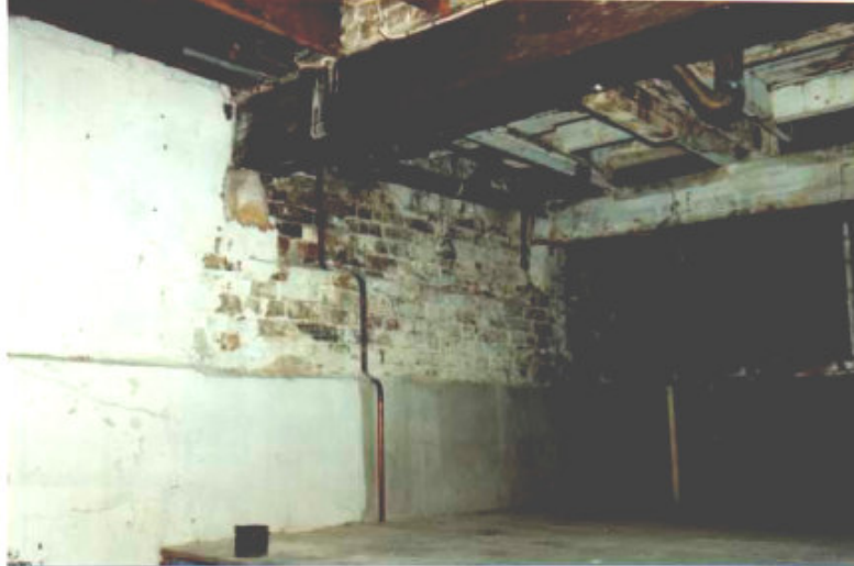
103 1 Top plate level of rear room that is now Room 0.6/0.8
