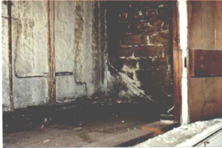
103 1 Stair landing roof plate over Room 1.2a
