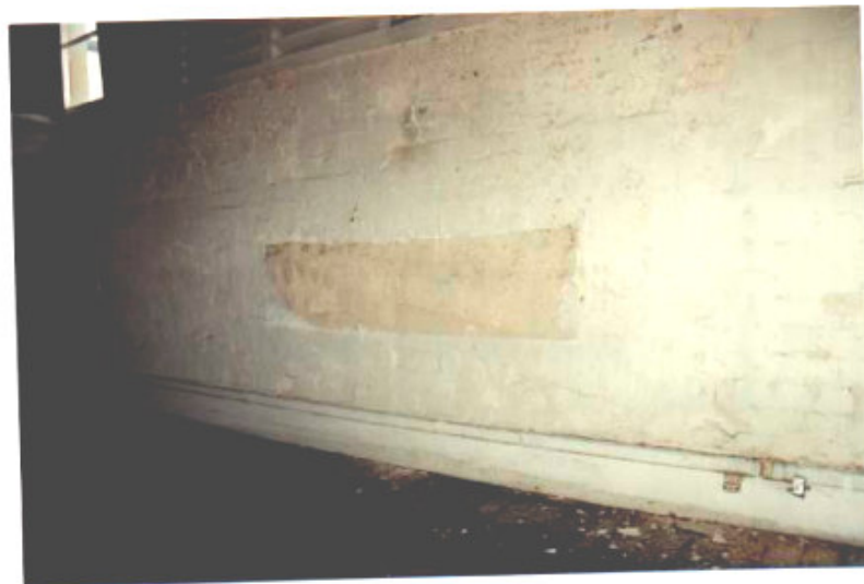
Closed in camber arch from earlier out building Room 1.4a
