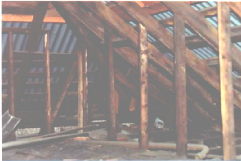
103 7 Timber floor and wall studs in attic over Room 2.6
