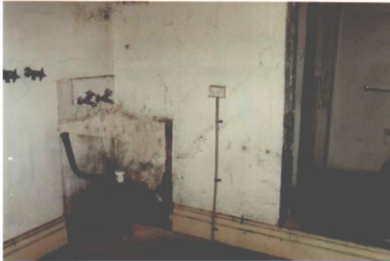
103.3 Impressions of original stair in Room1.6
