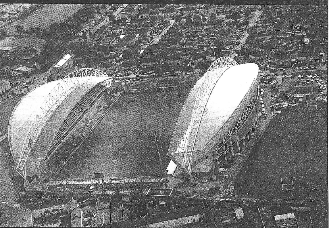
Ready for lift-off: An aerial view of the nearly completed Thomond Park taken this Tuesday ahead of the historic first match at the new stadium on Friday between Munster and Ulster Under 20s PICTURE: DERMOT LYNCH
