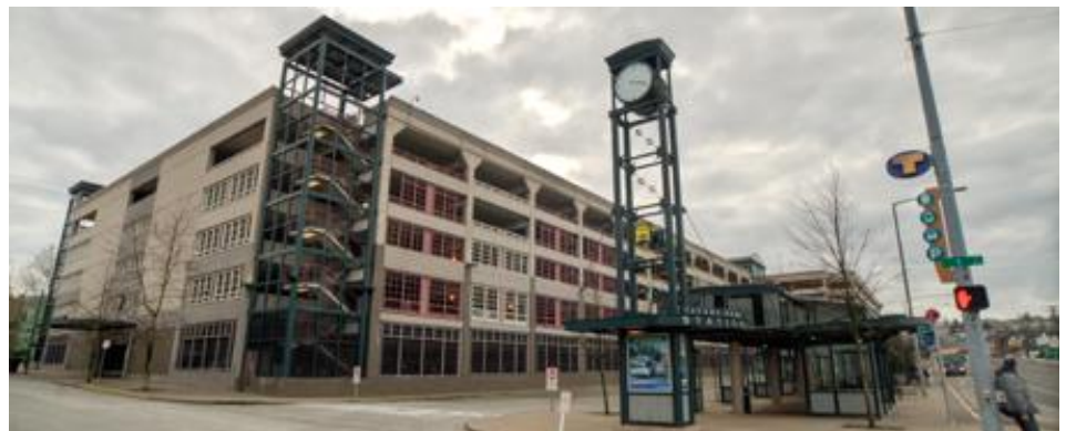
Figure 15: Tacoma Dome Station
