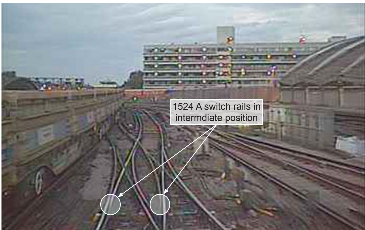
Figure 4: View from the train's forward facing CCTV of 1524 A points lying midway between normal (left switch rail closed) and reverse (right switch rail closed) (see appendix)
