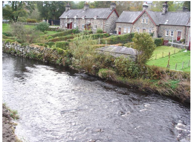
National Trust properties are protected by reinforced banks
