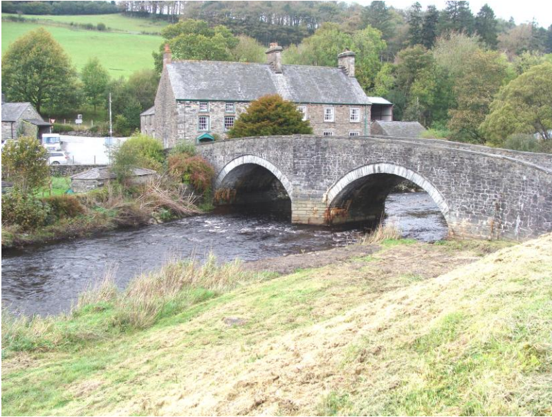
The bridge over the Conwy at the village of Ysbyty Ifan
