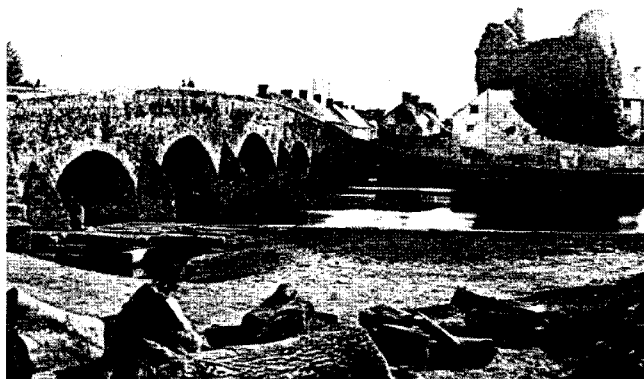
The bridge at Leighlinbridge
