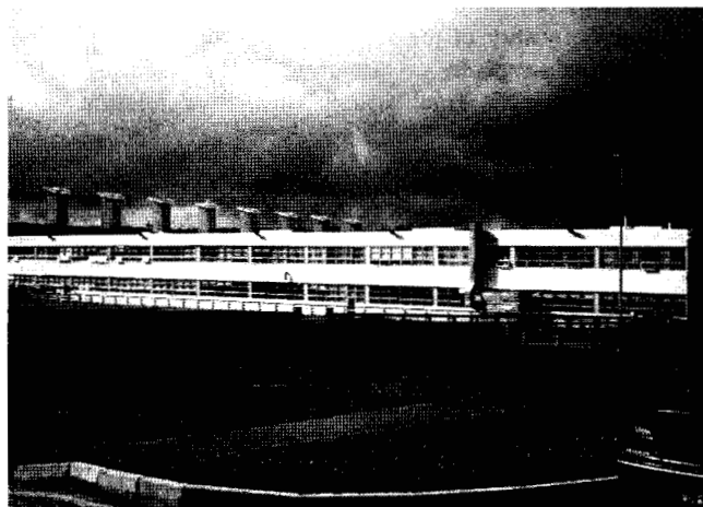
A rear view of the ITC after renovation in 2010
