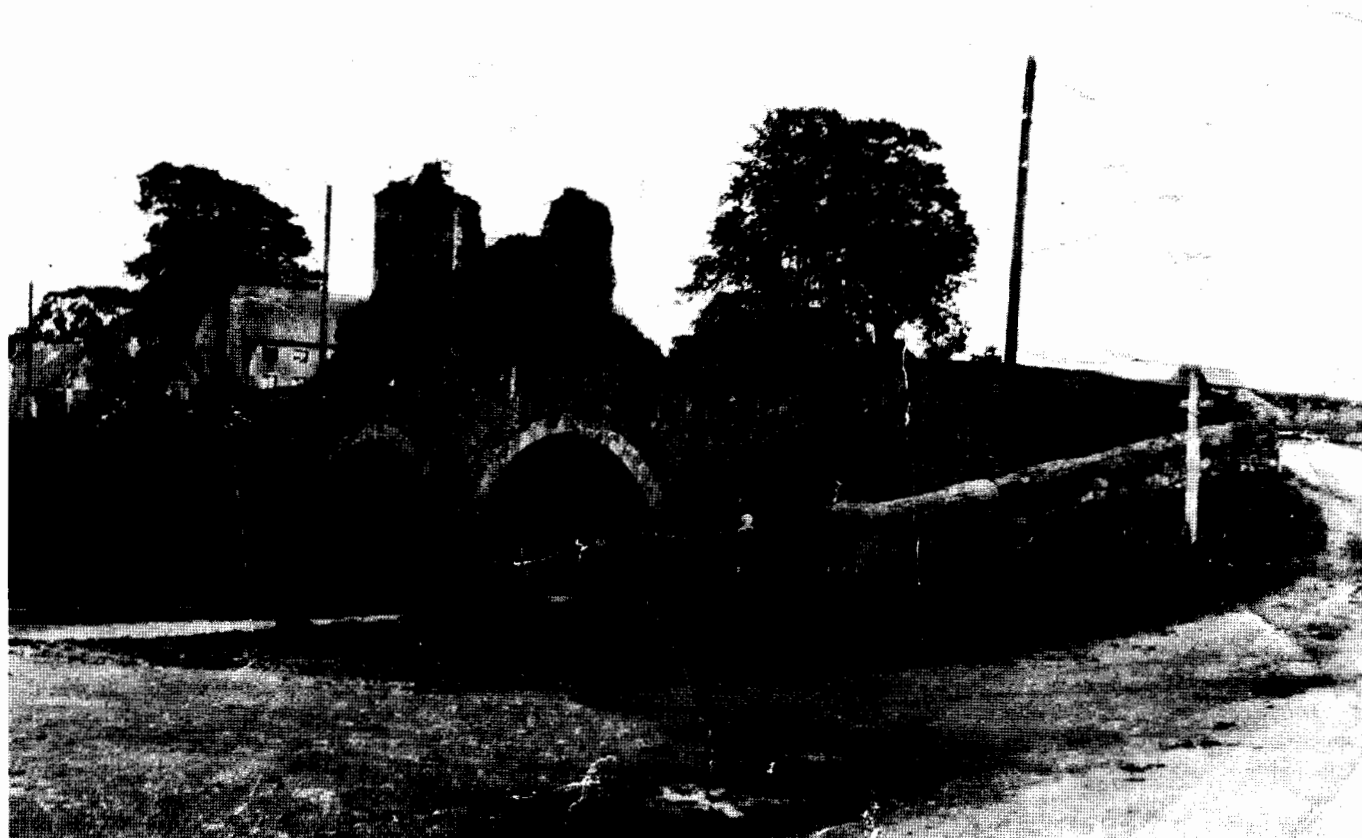
1940s view (looking south) of the bridge in Leighlin. Courtesy: Mr Jer Monaghan
