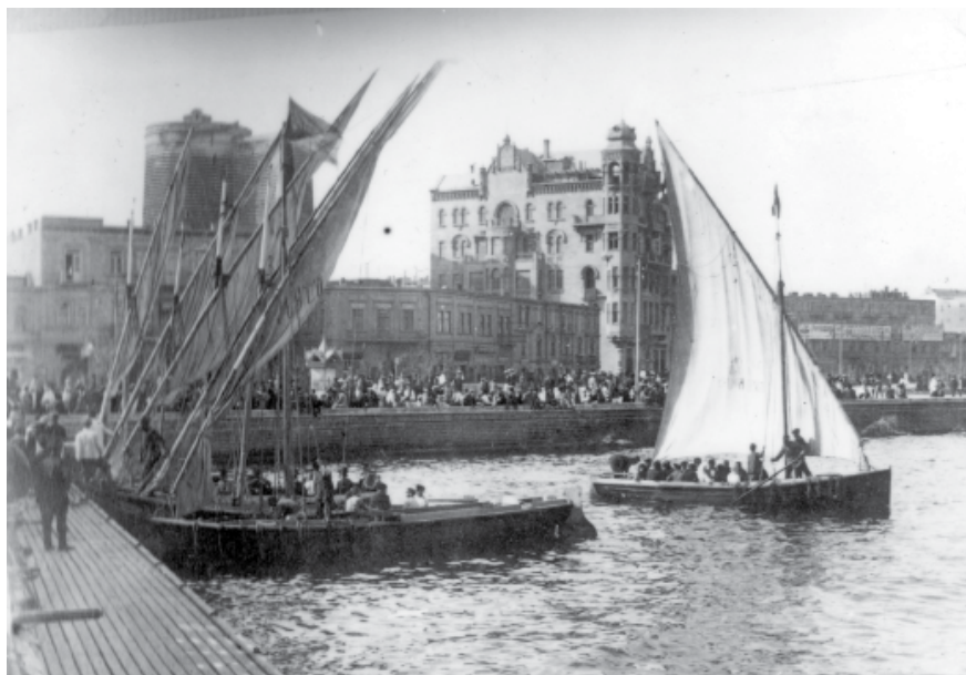
The Hajinski House on the Aleksandrovs Embankment
